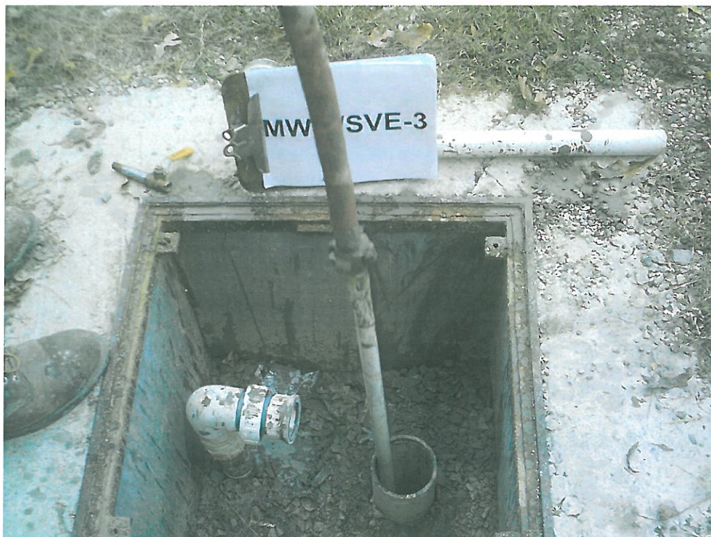
Photograph 8: Typical remediation system well during abandonment
