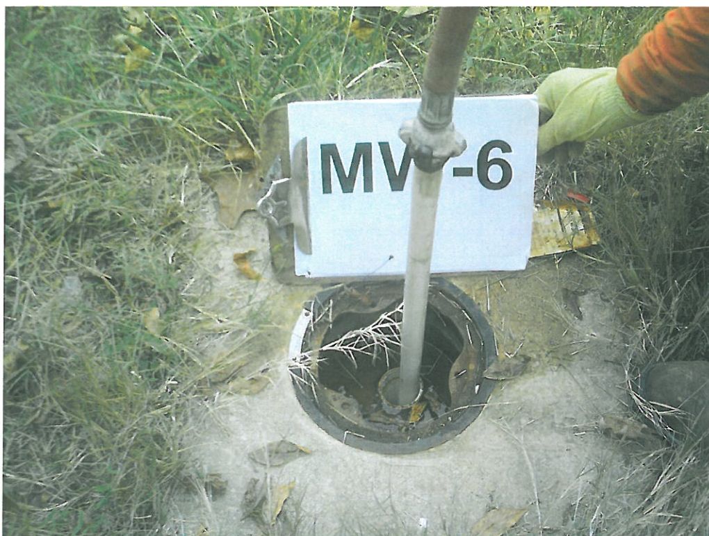
Photograph 5: Typical monitoring well during abandonment
