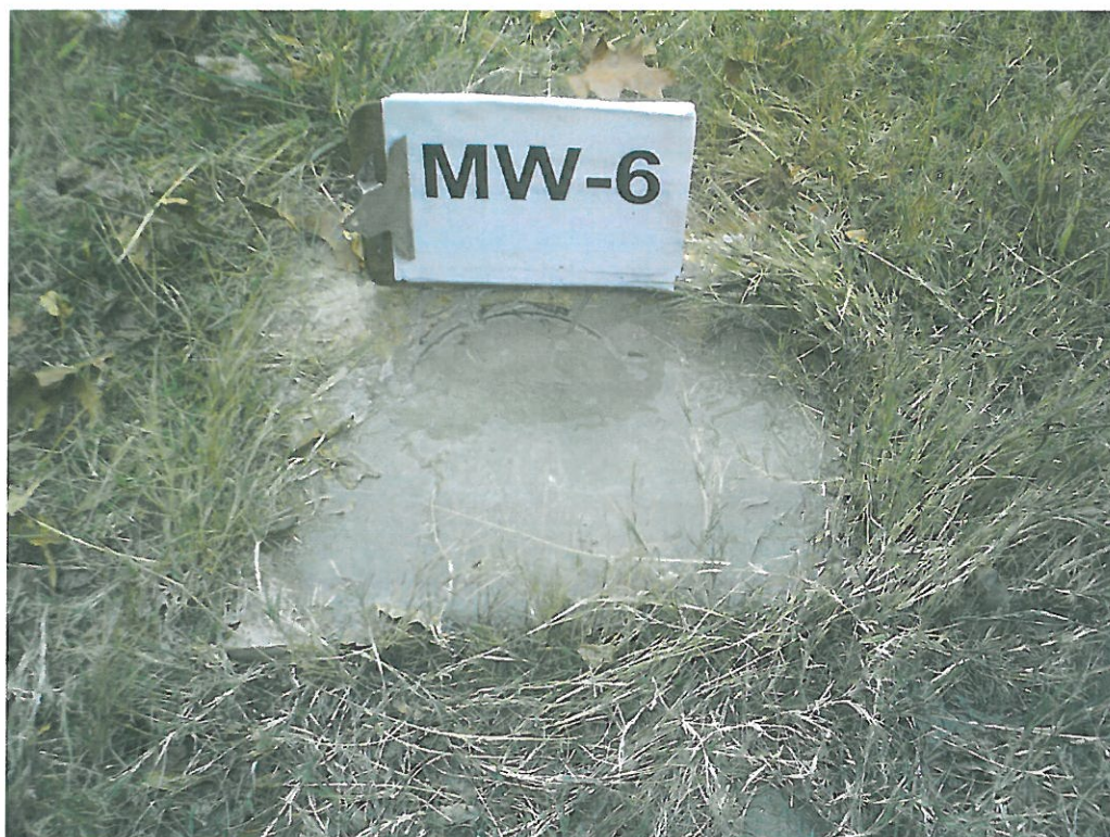
Photograph 6: Typical monitoring well during abandonment
