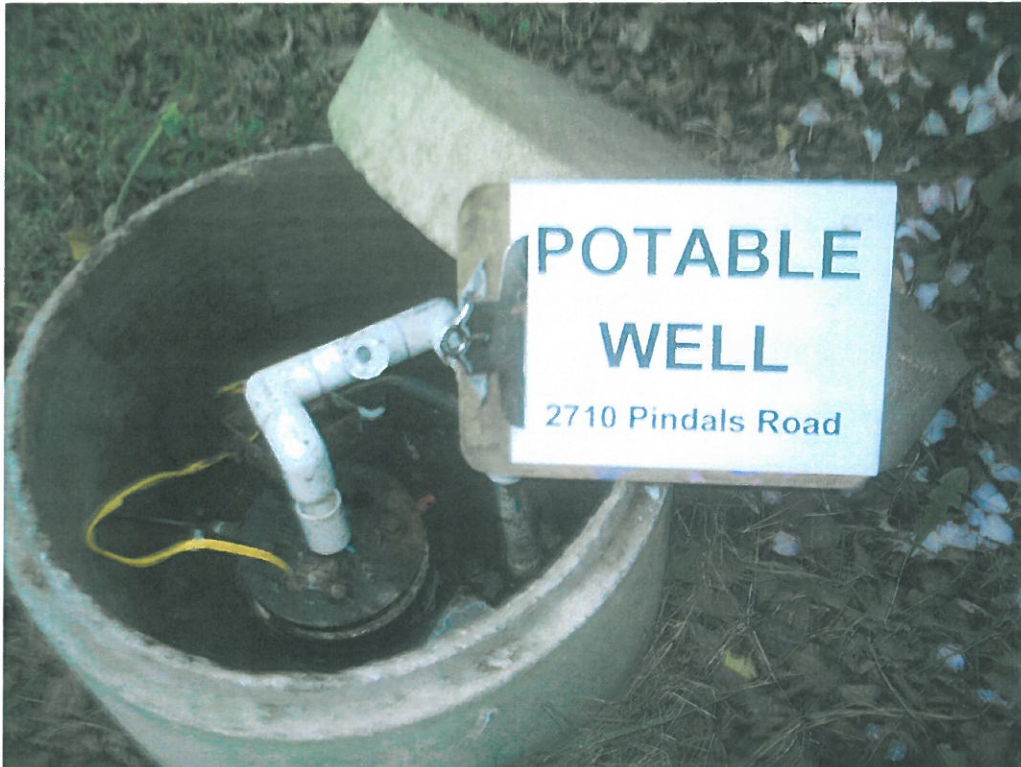
Photograph 1: Potable well at 2710 Pindals Road prior to abandonment
