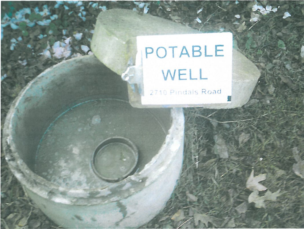
Photograph 3: Potable well at 2710 Pindals Road after abandonment
