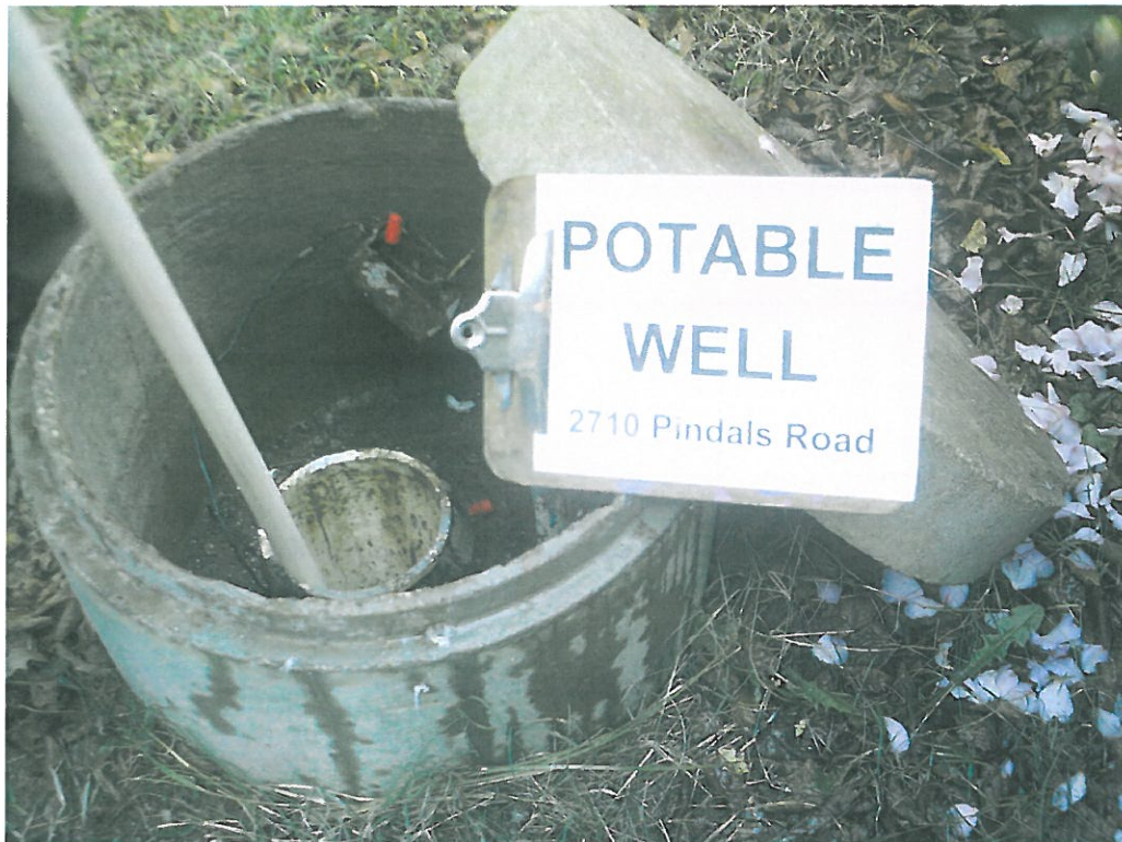
Photograph 2: Potable well at 2710 Pindals Road during abandonment
