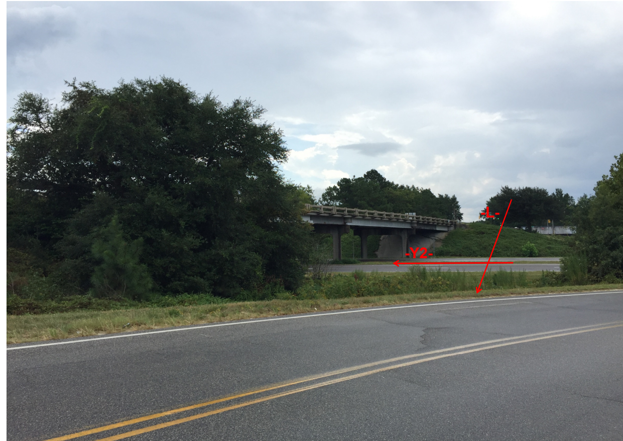
View Looking West from East of End Bent 2
