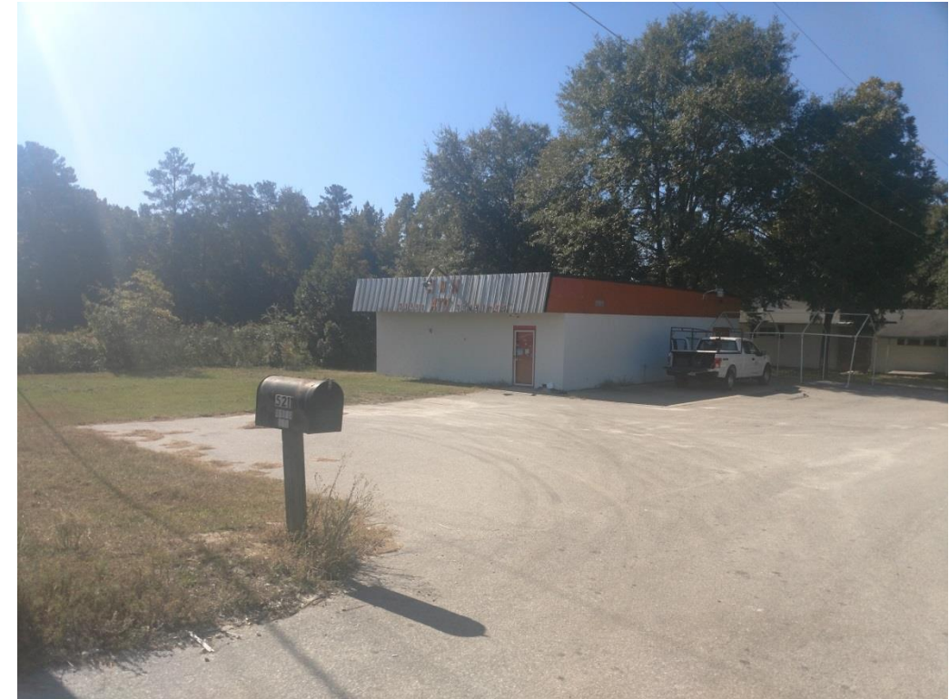
b. Photo from north side of site looking south.
