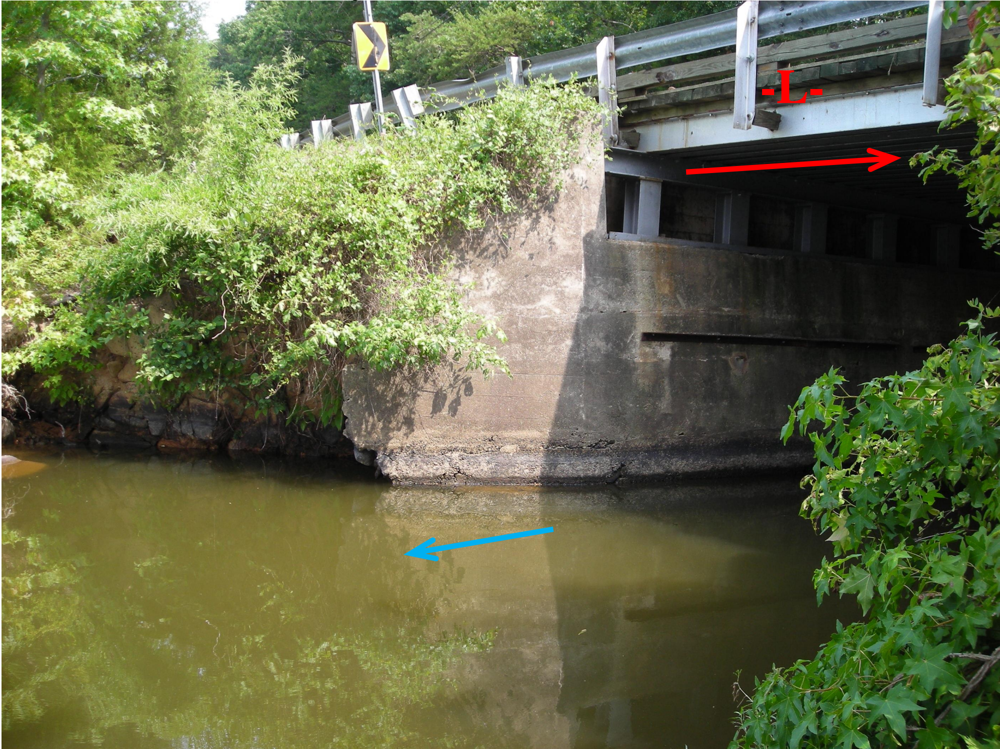
Bridge No. 20 on -L- (SR 1616) over Dial Creek
