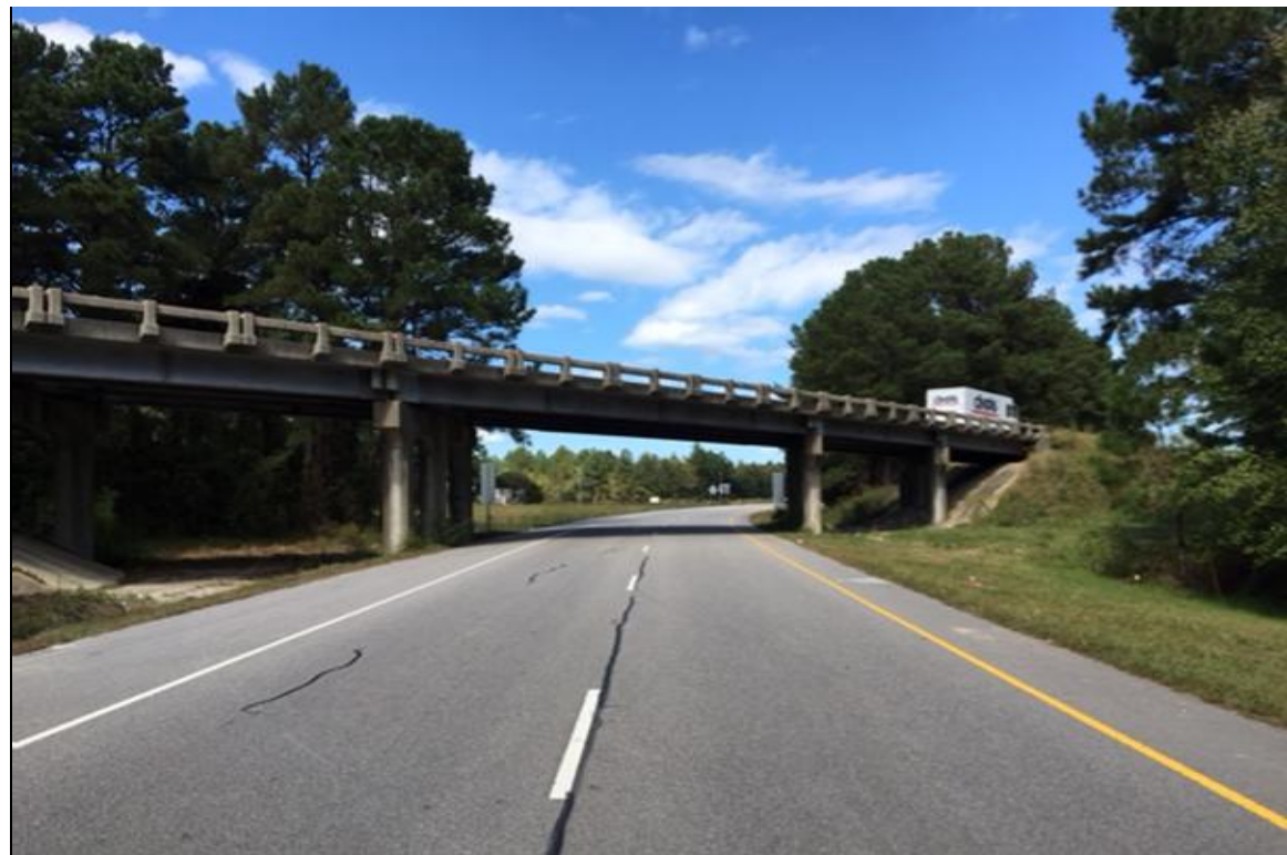
PHOTOGRAPH NO. 2: ON -L2- ALIGNMENT, SOUTH OF -L- ALIGNMENT, LOOKING NORTH
