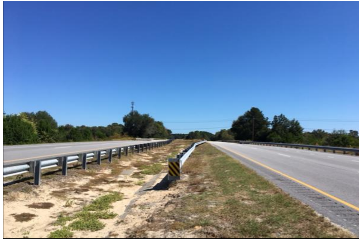
PHOTOGRAPH NO. 1: WEST APPROACH TO END BENT NO. 1 BETWEEN -L1- AND -L2- ALIGNMENTS, LOOKING EAST
