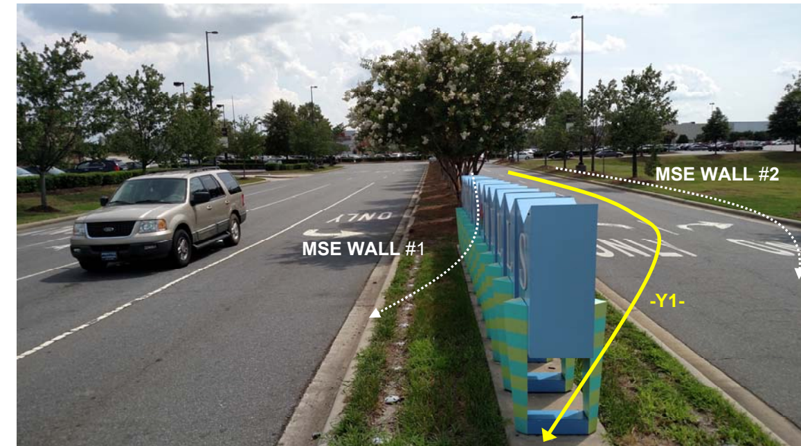
Photograph No. 3: On -Y1- (Kings Grant Pavilion) looking southwest
