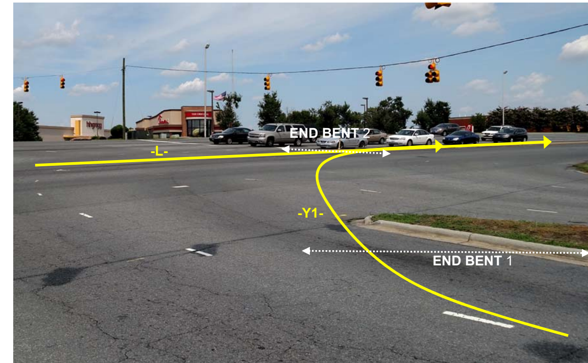
Photograph No. 4: Looking northeast towards End Bent 2
