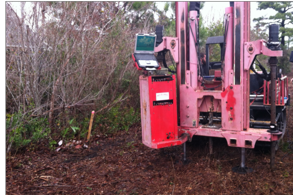
CPT RIG AT STAKED B-2 LOCATION
