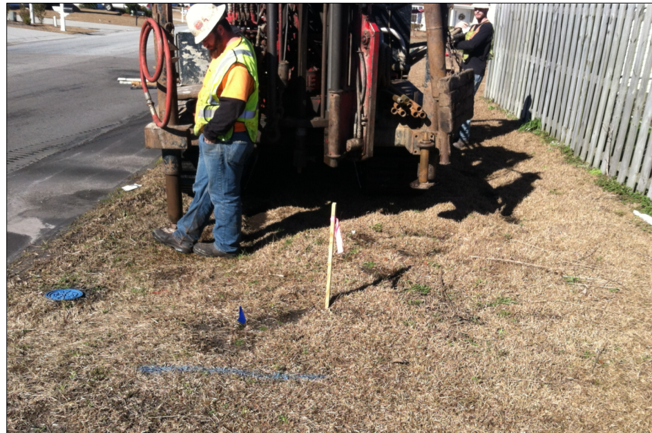
SPT RIG AT STAKED B-1 LOCATION
