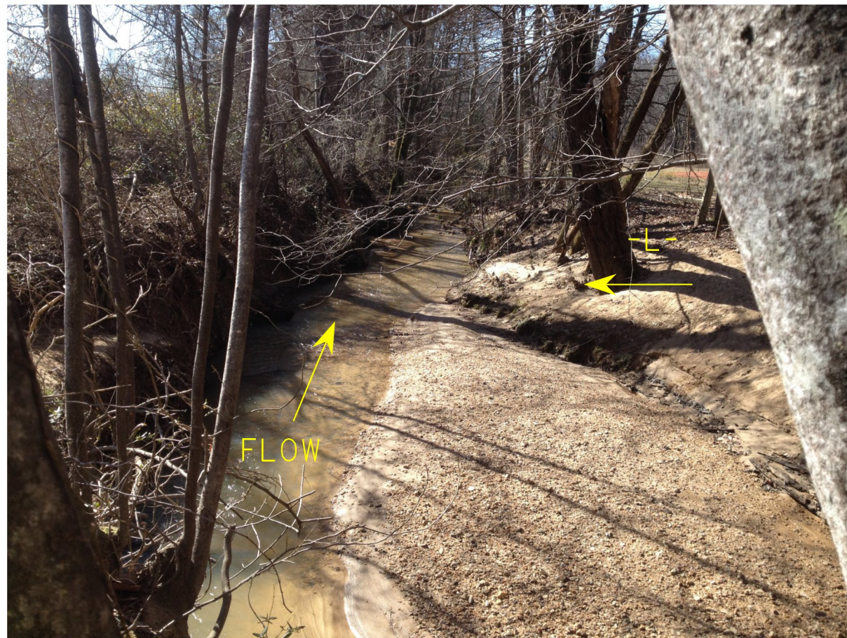
Looking south along Lowery Mill Creek between Bent 1 and Bent 2
