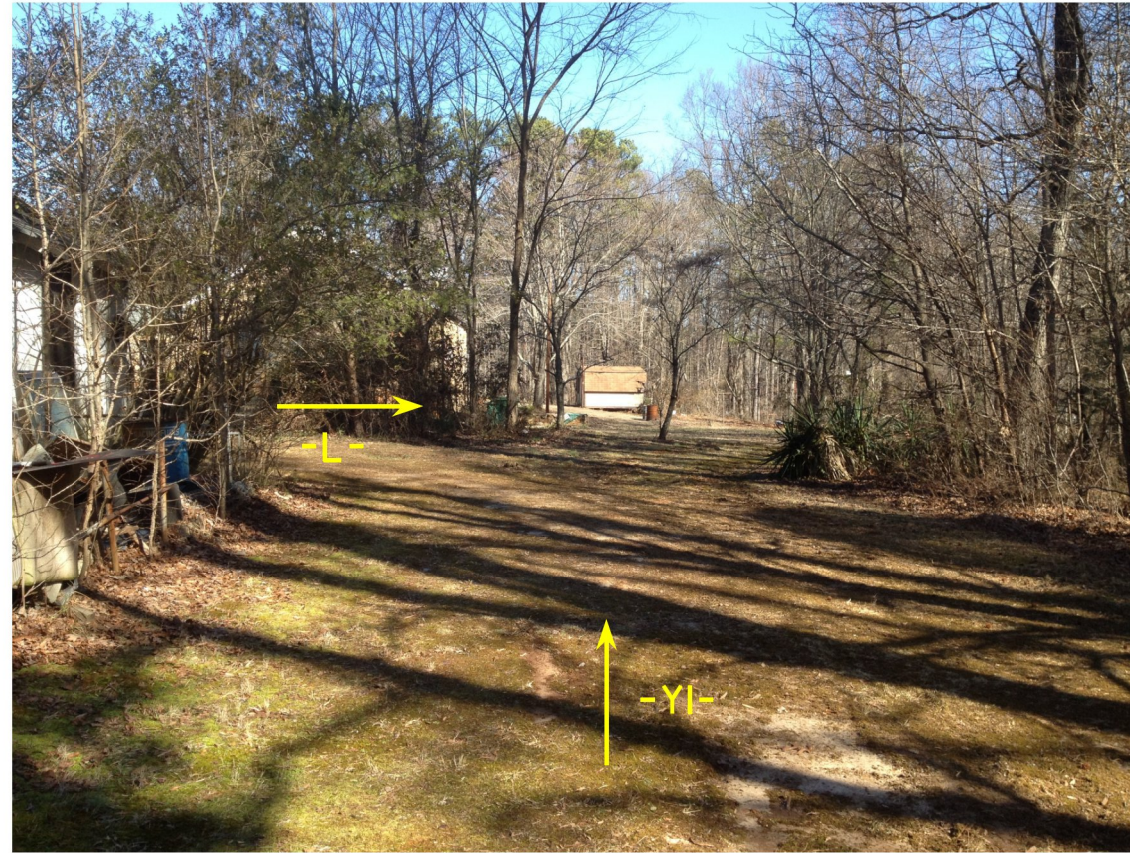
Site Photo No. 1: End Bent 1 -YI- (US 311) Looking Upstation (North)
