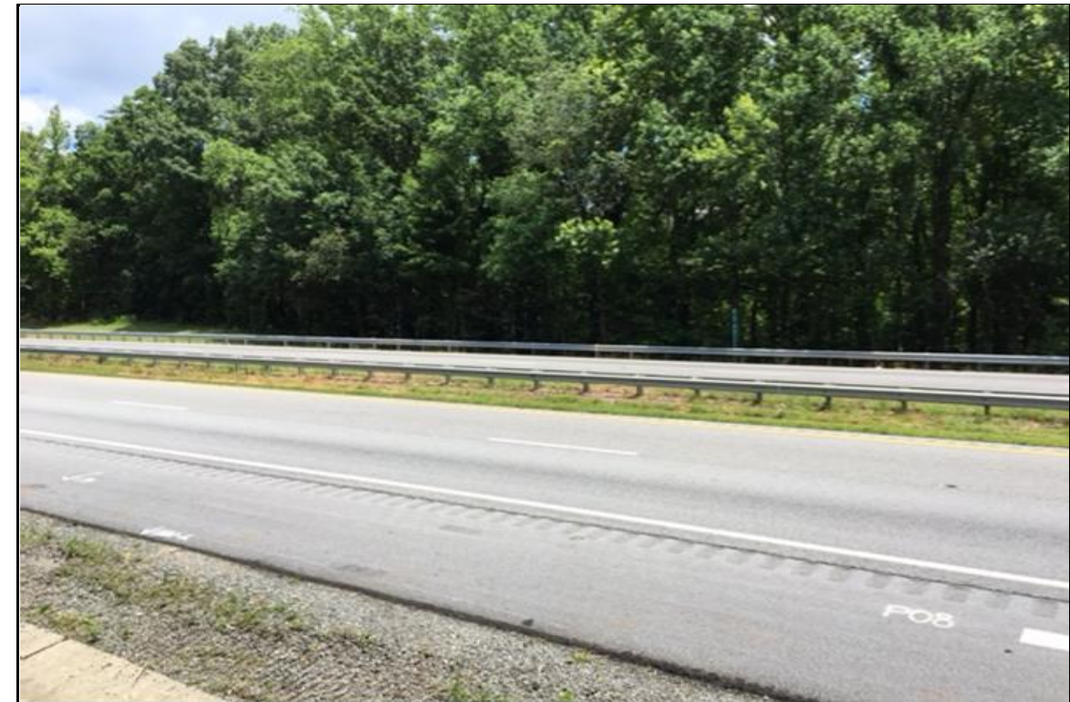
PHOTOGRAPH NO. 4: SOUTH APPROACH TO END BENT NO. 2 ON -RP_F- ALIGNMENT, LOOKING NORTH
