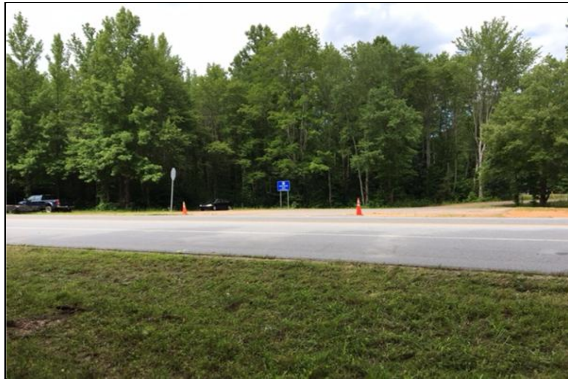
PHOTOGRAPH NO. 1: SOUTH APPROACH TO END BENT NO. 1 ON -RP_E- ALIGNMENT, LOOKING NORTH
