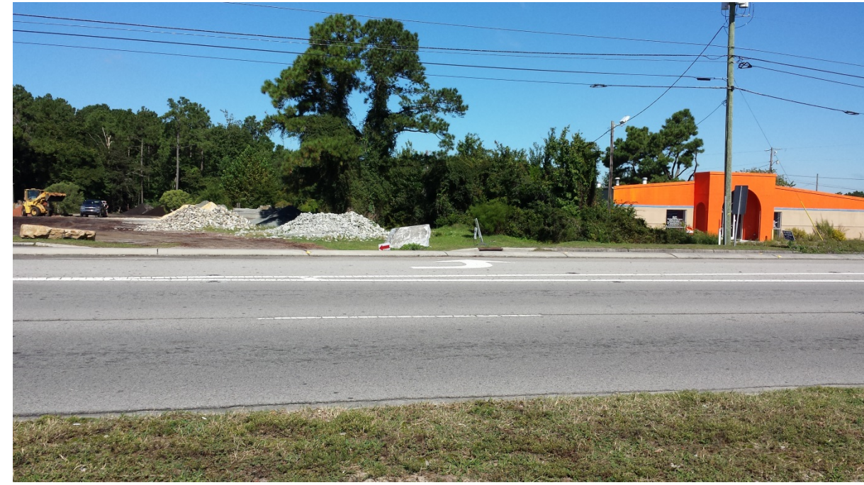
Photograph No. 3: View looking NW across Market Street from End Bent 1 toward End Bent 2
