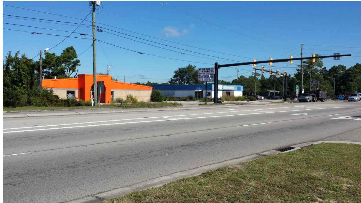
Photograph No. 1: View looking North across Market Street from End Bent 1 toward End Bent 2
