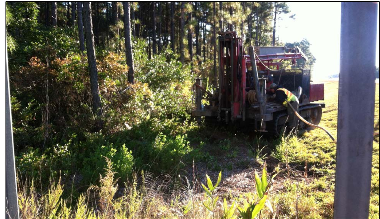
LOOKING LEFT TOWARDS -L-: DRILL RIG SETUP ON EB2-B
