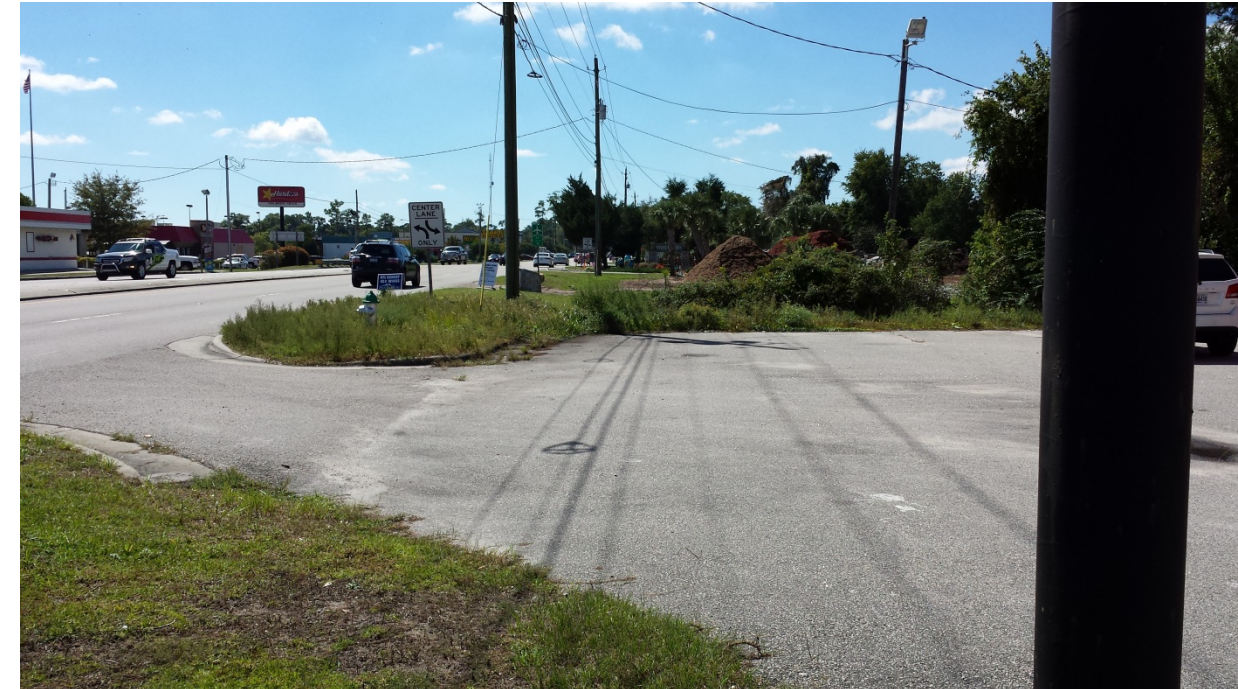
Photograph No. 4: View looking SW along End Bent 2, Market Street to left
