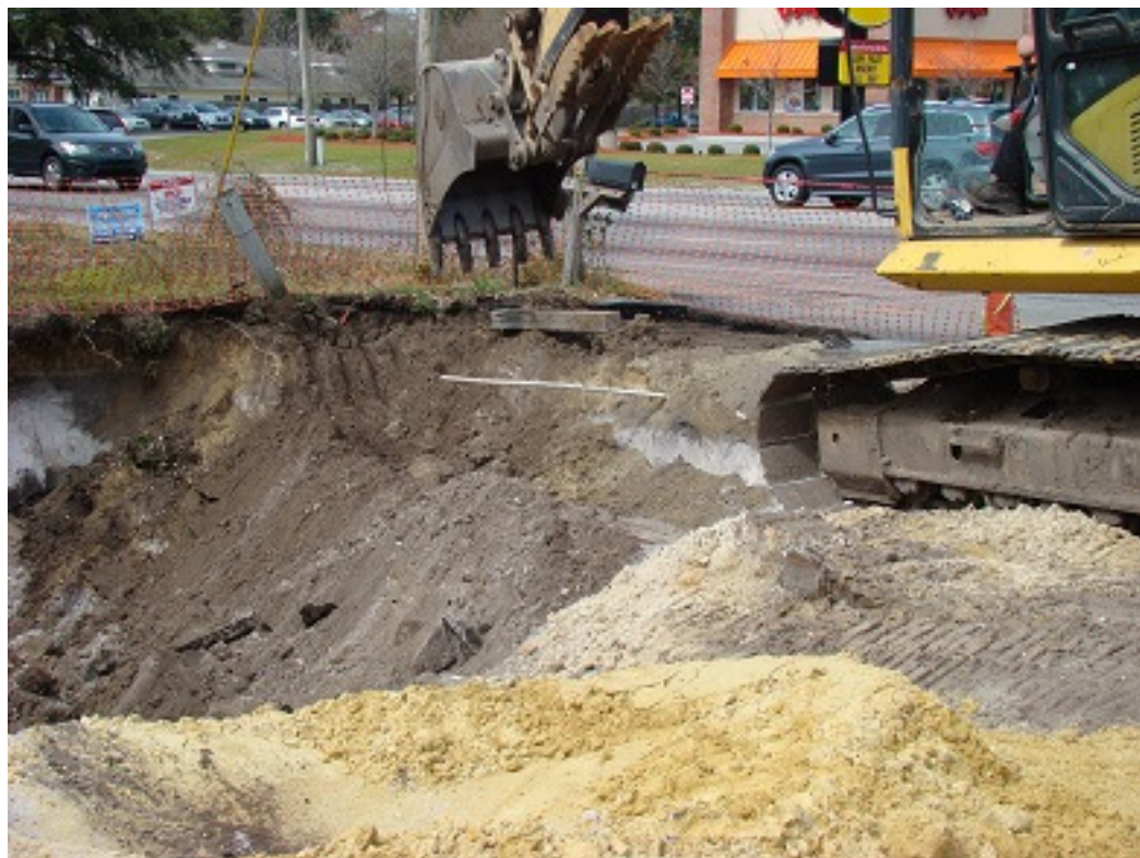
Photo 12: Begin over- excavation near MW- 5, facing west
