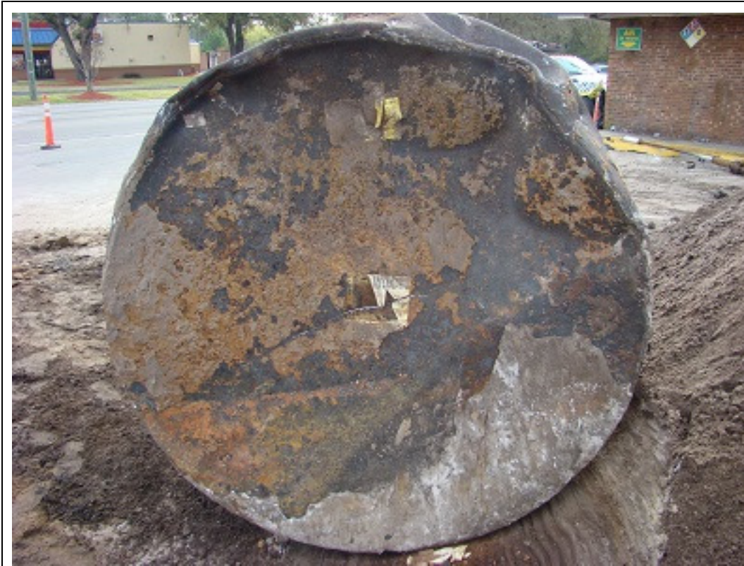
Photo 11: End view of UST #3
