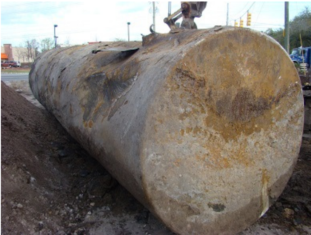
Photo 10: Side and end view of UST #3
