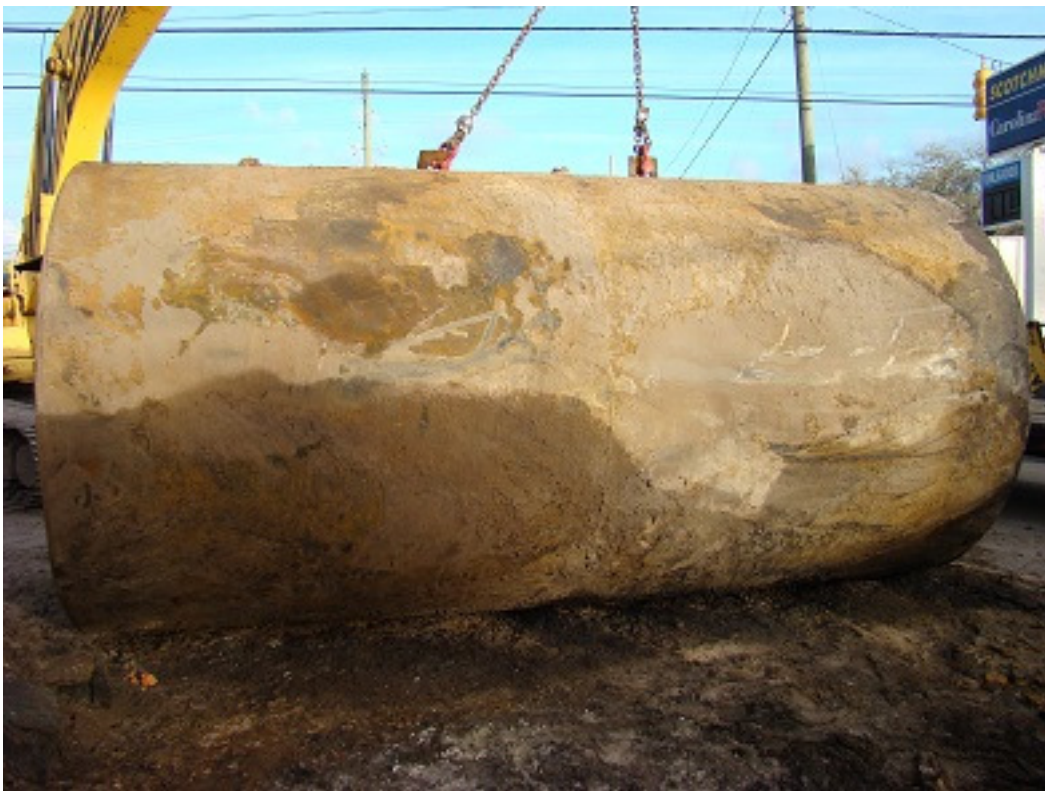
Photo 8: Side view of UST #2
