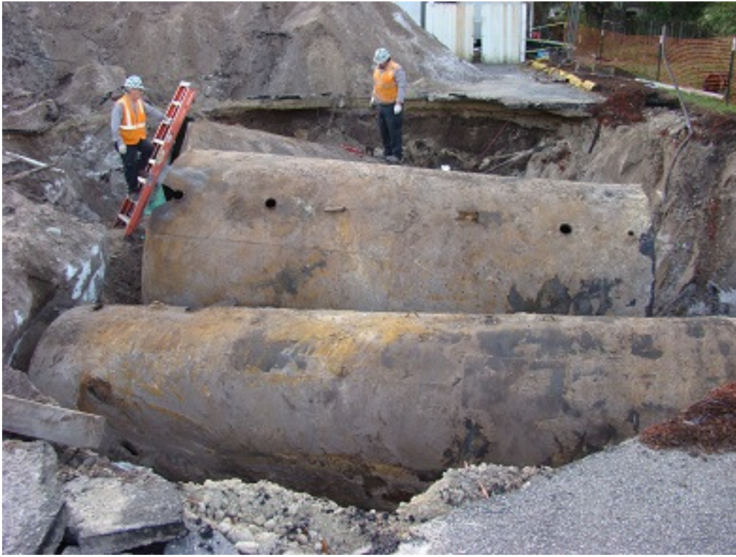
Photo 1: USTs uncovered and cleaned, facing southeast
