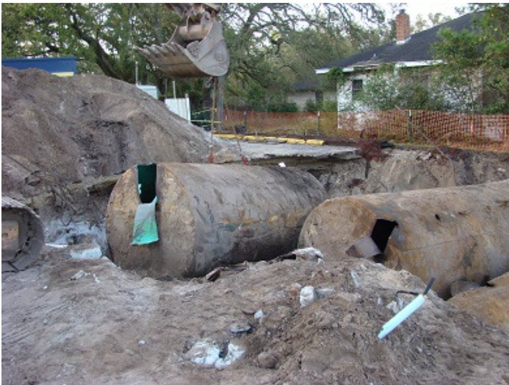
Photo 2: Removing UST #2- 6,000 gallon UST facing south
