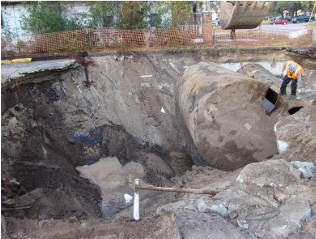
Photo 3: Removing UST #1- 6,000 gallon UST facing southwest
