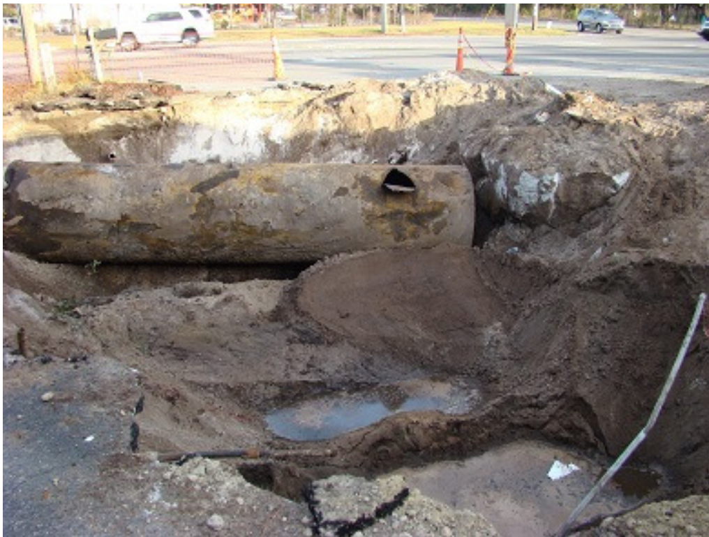
Photo 4: Removing UST #3 – 4,000 gallon UST facing north
