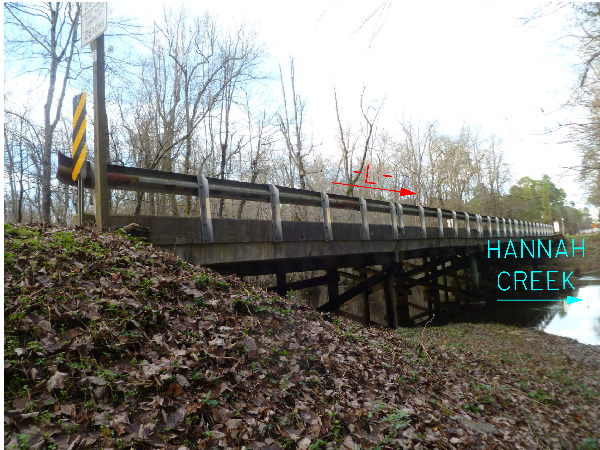
LOOKING NORTH TOWARDS END BENT 2
