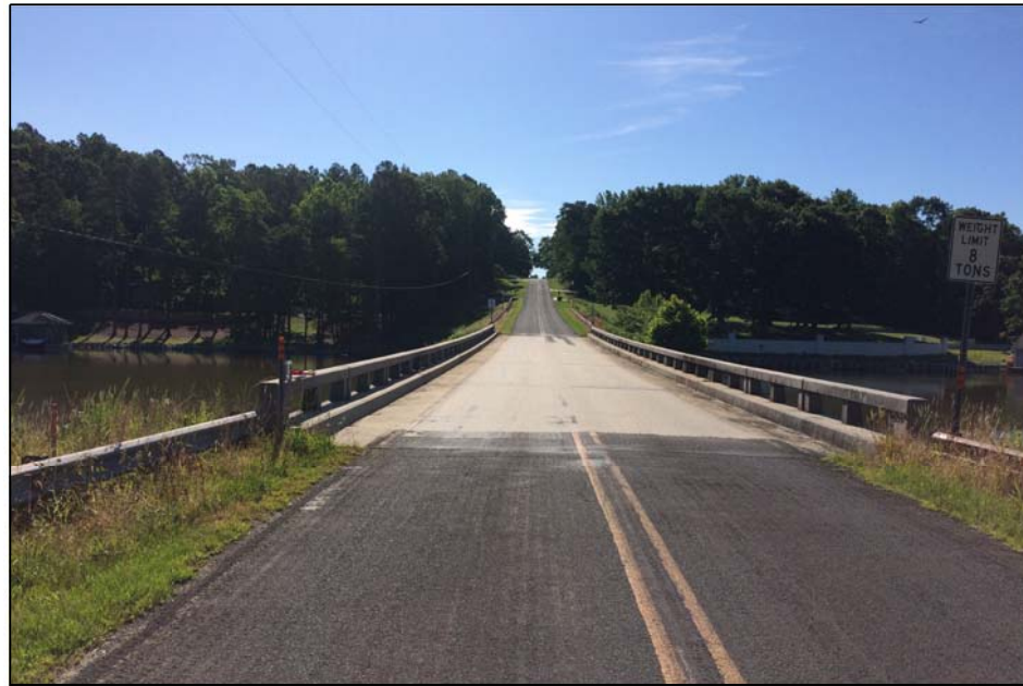
LOOKING UPSTATION ALONG -L-
