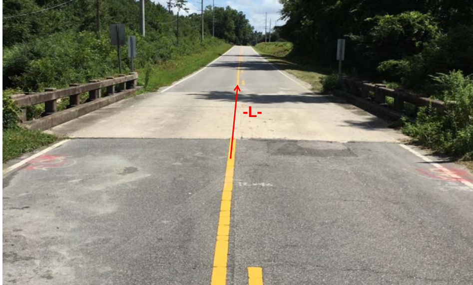
View Looking North along -L- from End Bent 1
