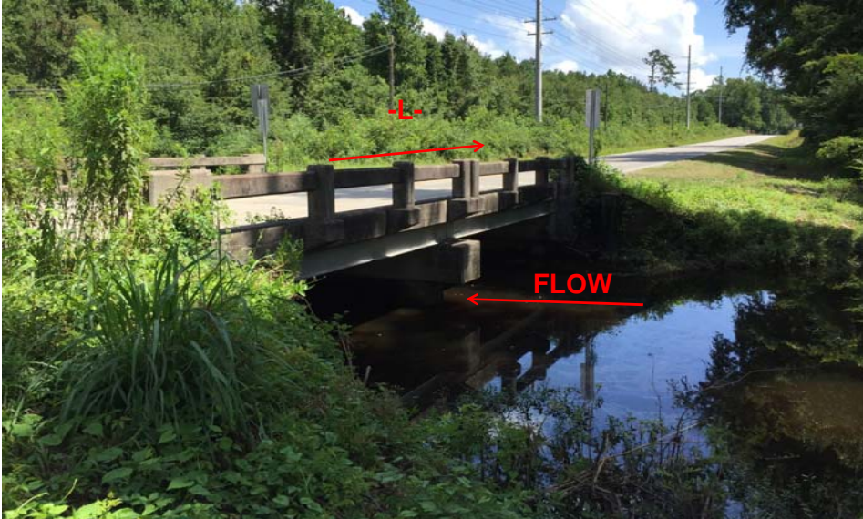
Profile of Bridge From Northwest of End Bent 1
