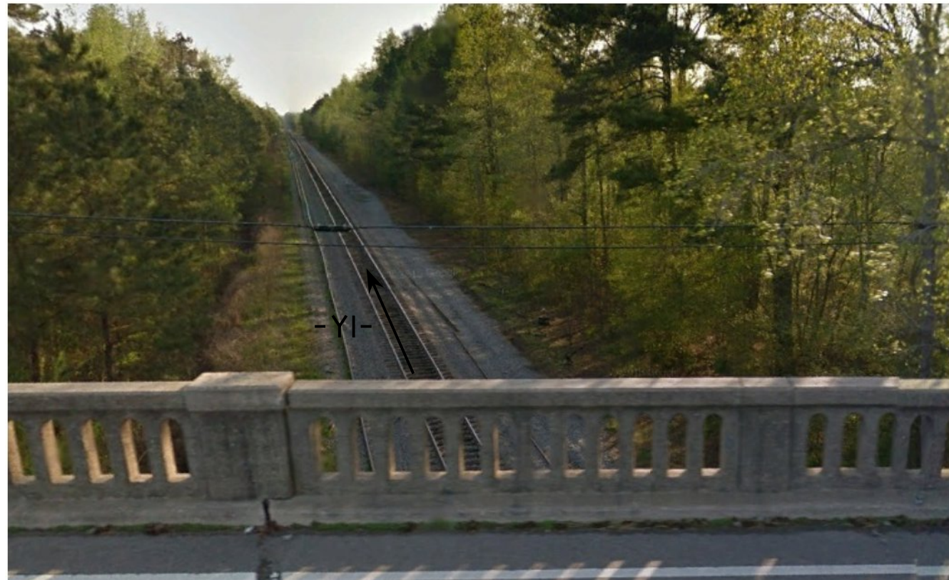
Site Photo No. 1: -YI- (CSX RR) Looking Upstation (West)
