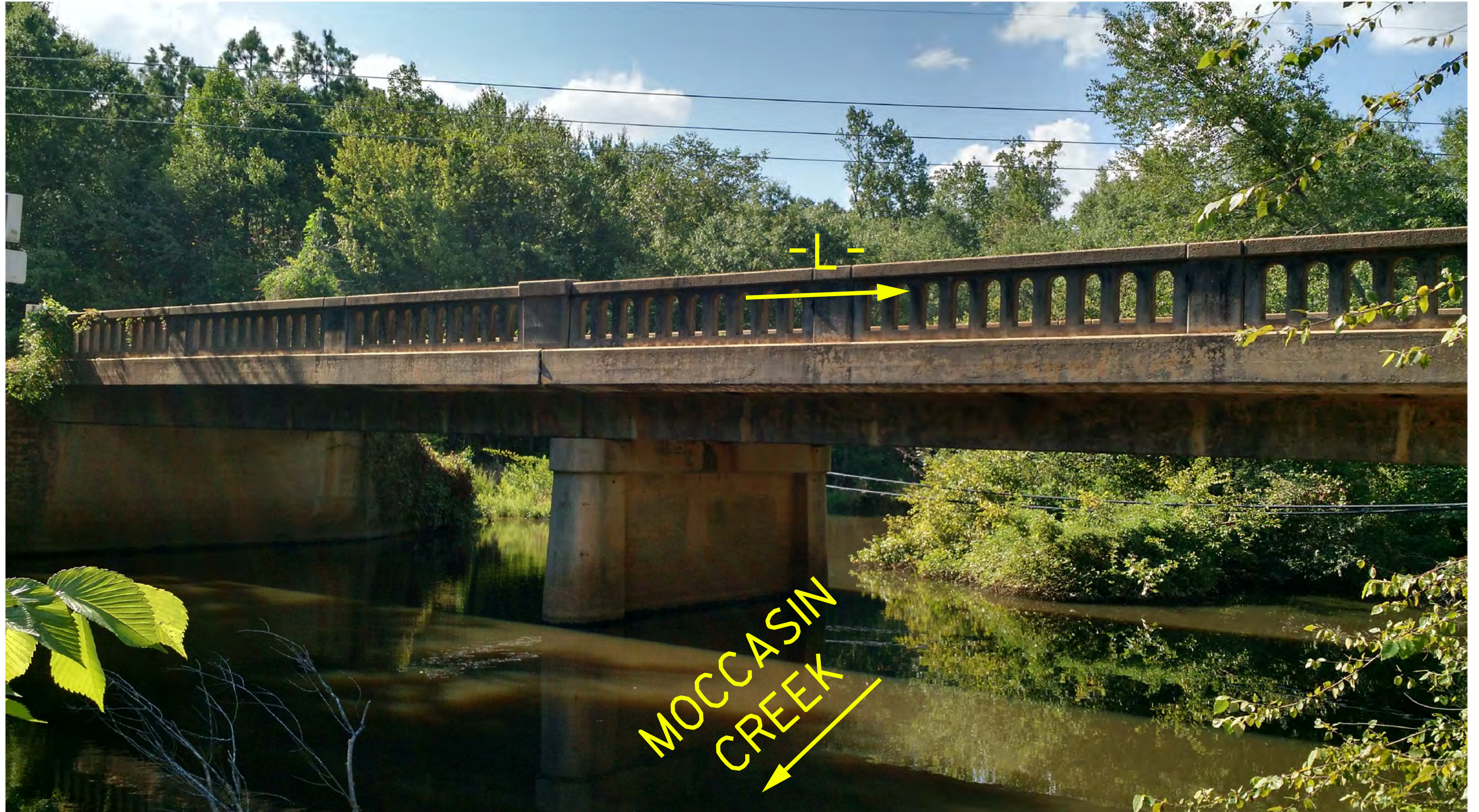
LOOKING NORTH AT BRIDGE NO. 20
