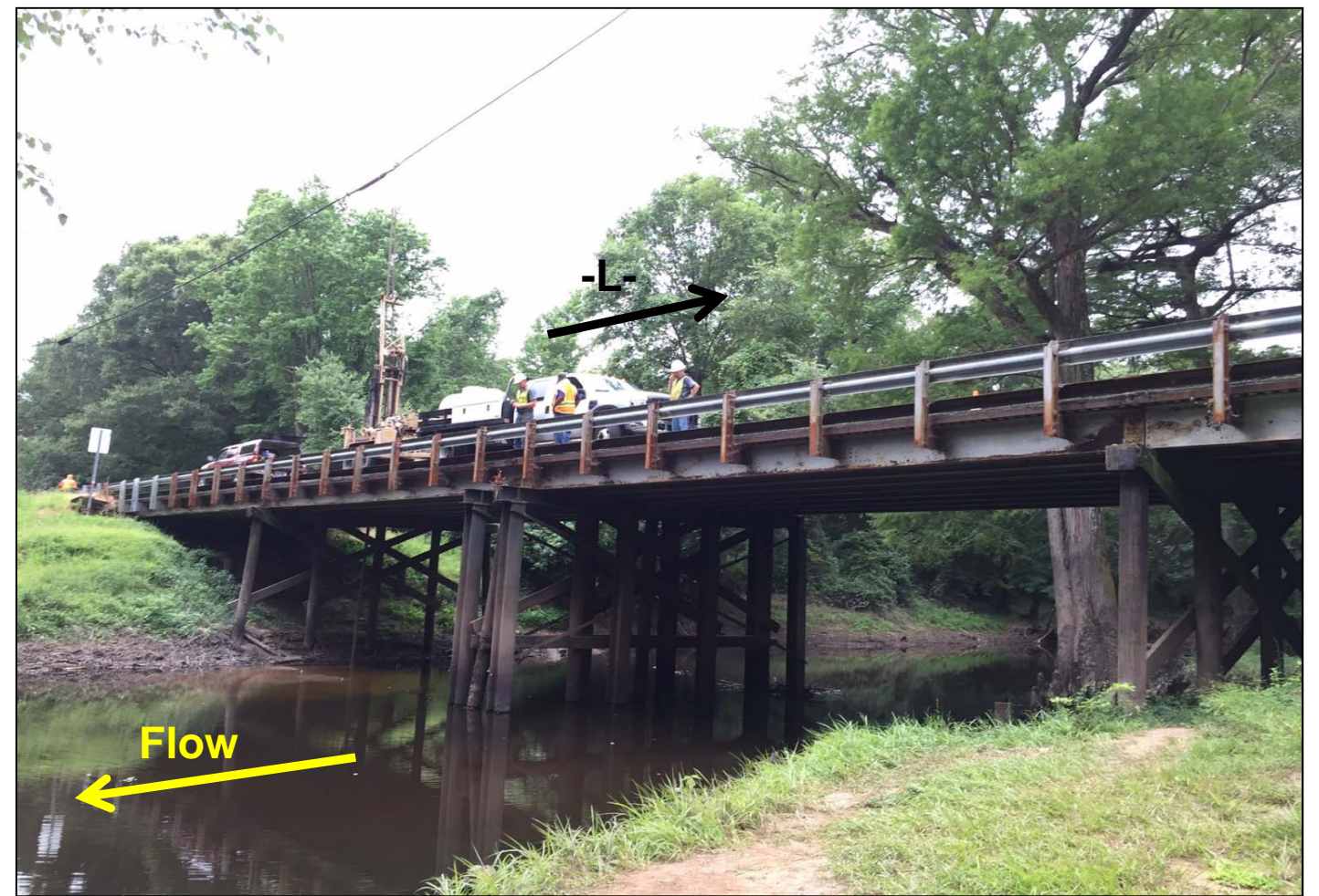
View of Bridge No. 11 looking southwest
