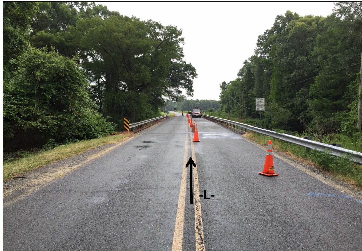
View of SR 1201 looking northeast
