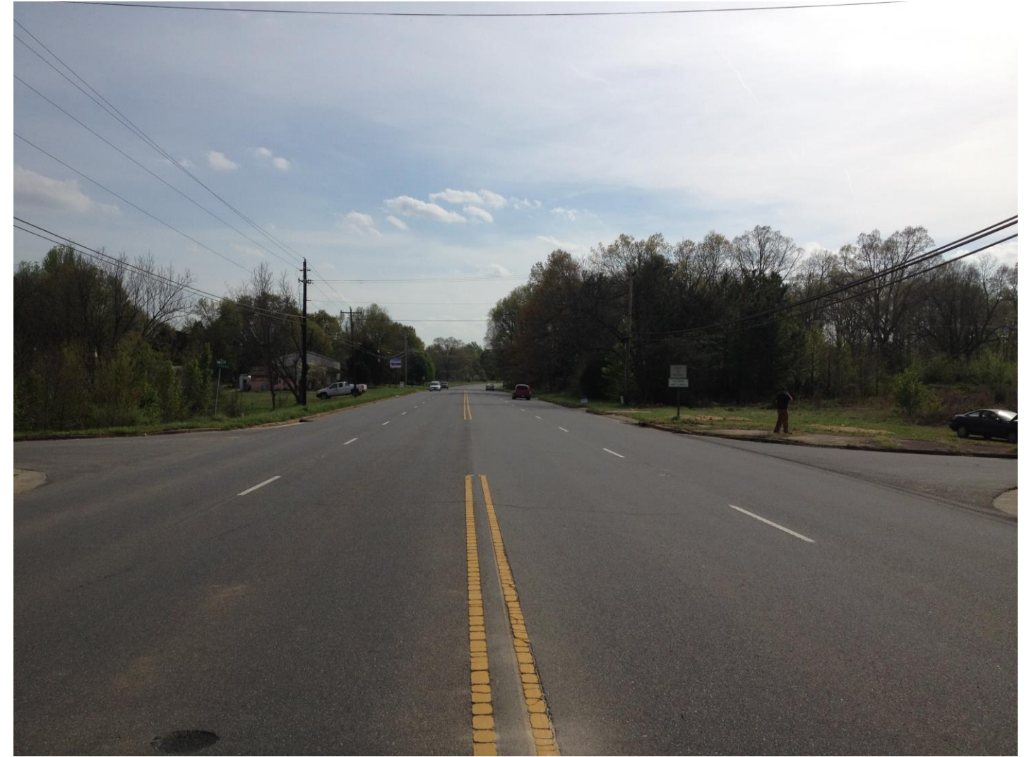
Standing at the centerline of -Y9- at End Bent 1 looking South
