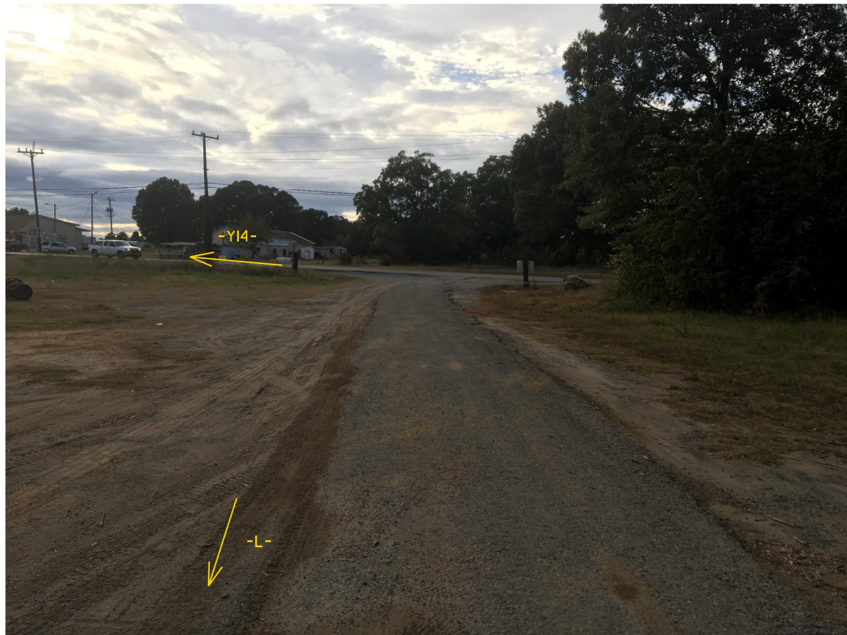
PHOTO NO. 2: -L- LOOKING DOWNSTATION (NORTH) AT END BENT NO. 2
