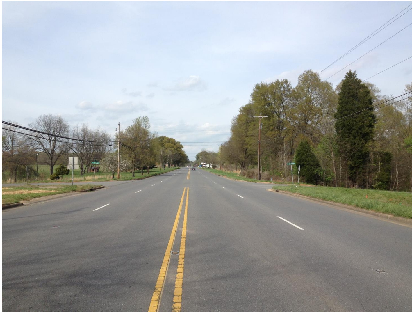
Standing at the centerline of -Y9- at End Bent 2 looking North
