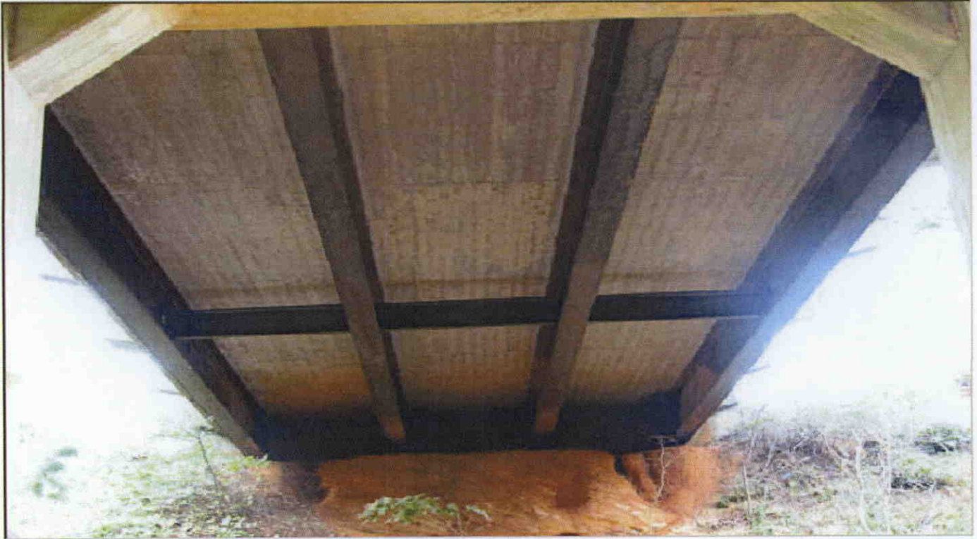
TYPICAL END BENT
