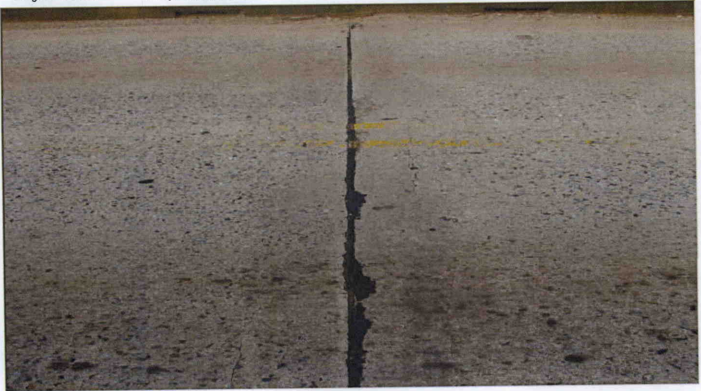
JOINT OVER INTERIOR BENT
