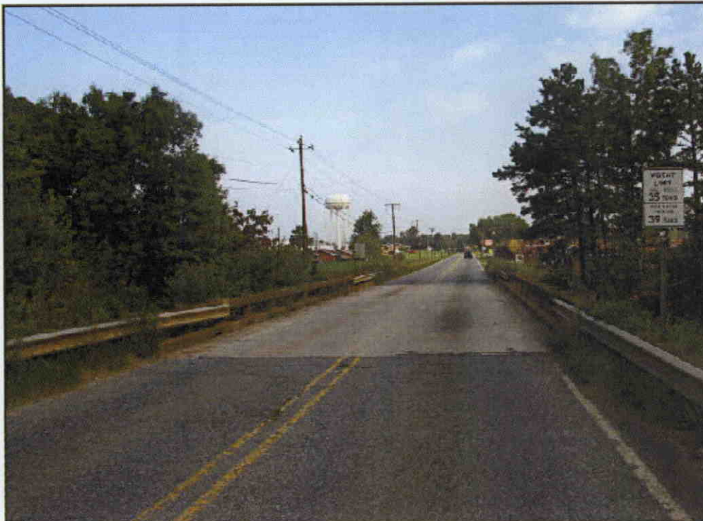
Photo Looking LOOKING NORTH
