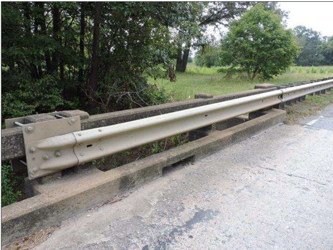
GUARDRAIL TO BARRIER RAIL TRANSITION AT SOUTHEAST CORNER, OTHERS SIMILAR
