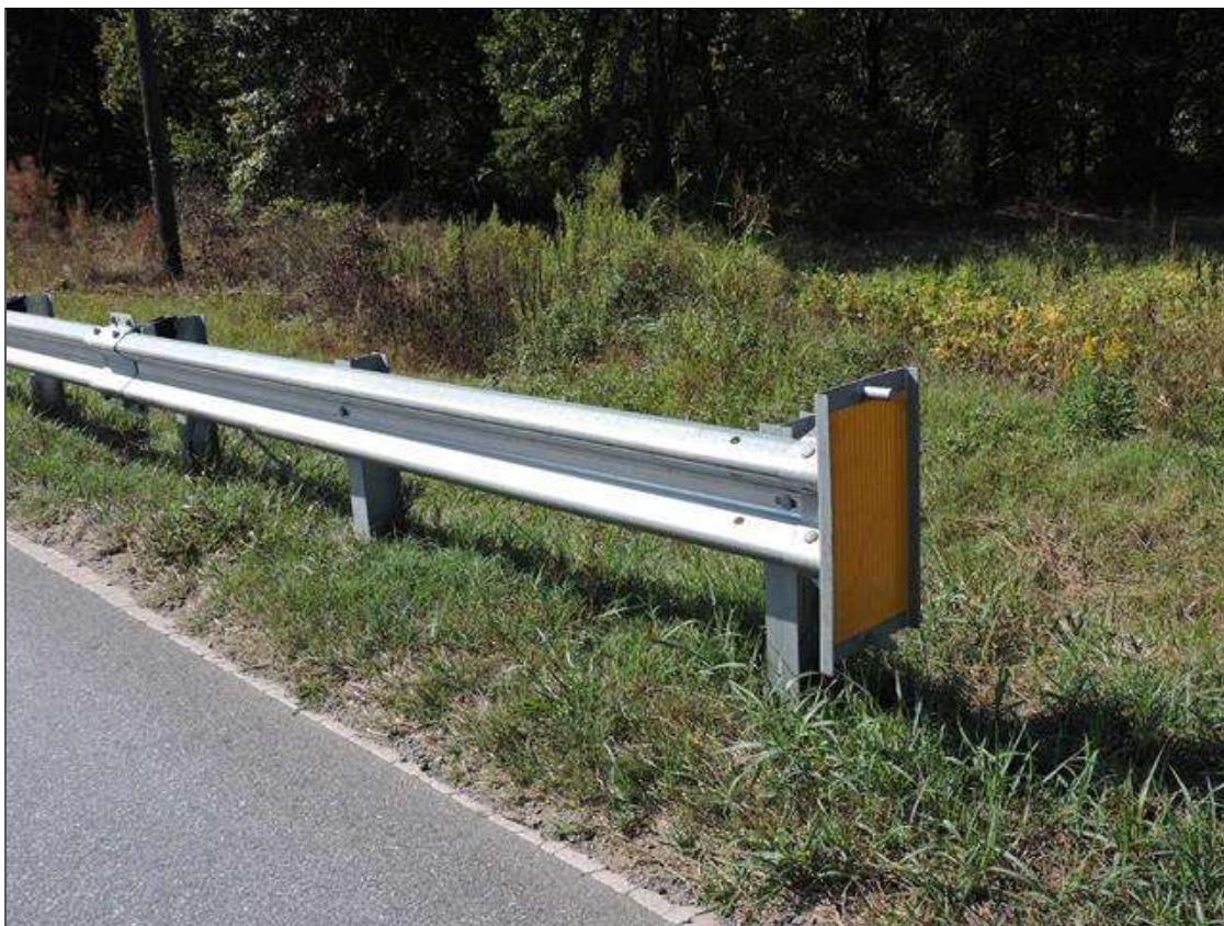
GUARDRAIL END TREATMENT AT NORTHWEST CORNER
