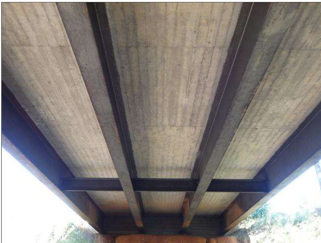
SPAN 2 UNDERDECK, SPAN 1 SIMILAR
