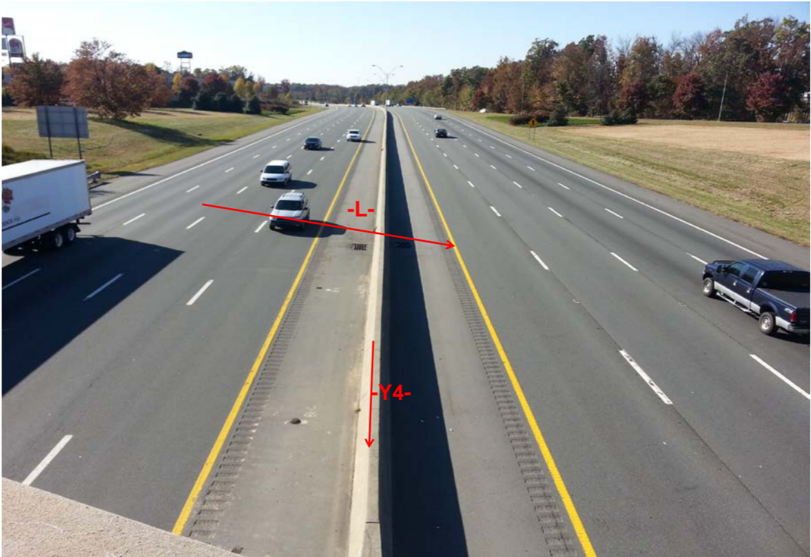
Profile of Bridge From Existing Bridge Looking West
