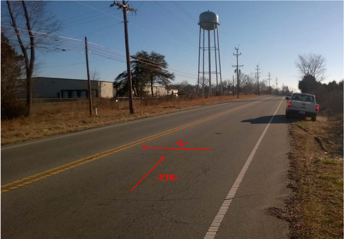
View Looking East along -Y16- from Bent No. 3
