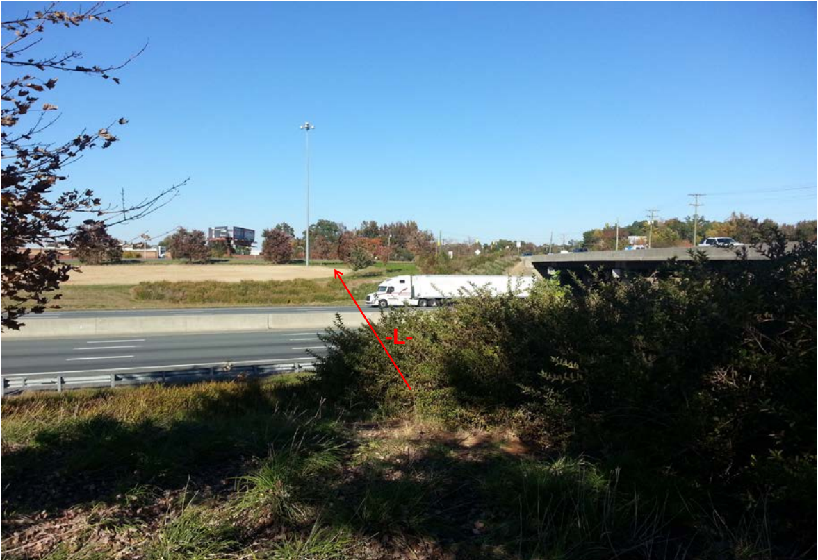
View Looking North along -NBL- from End Bent 1
