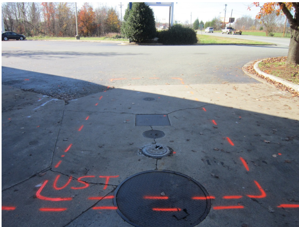
Parcel 21 (Spirit Master Funding In., LLC Property), looking southwest. Photo shows approximate marked location of Known UST No. 2 near the northwest corner of the canopy on Parcel 21.
