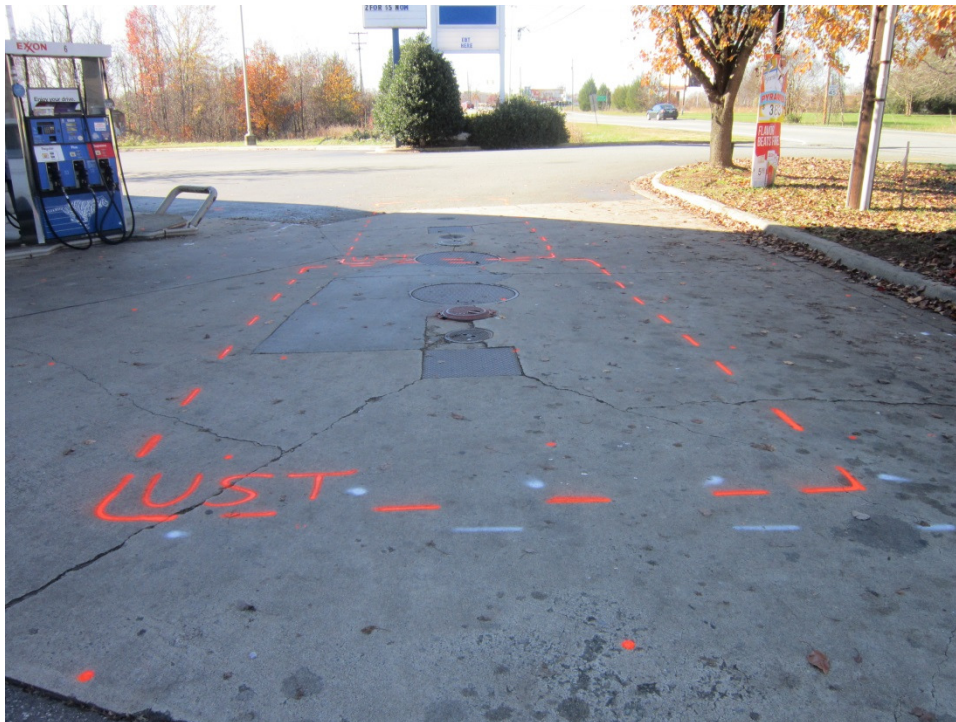
Parcel 21 (Spirit Master Funding In., LLC Property), looking southwest. Photo shows approximate marked location of Known UST No. 1 (foreground) and Known UST No. 2 (background) near the northwest corner of the canopy on Parcel 21.
