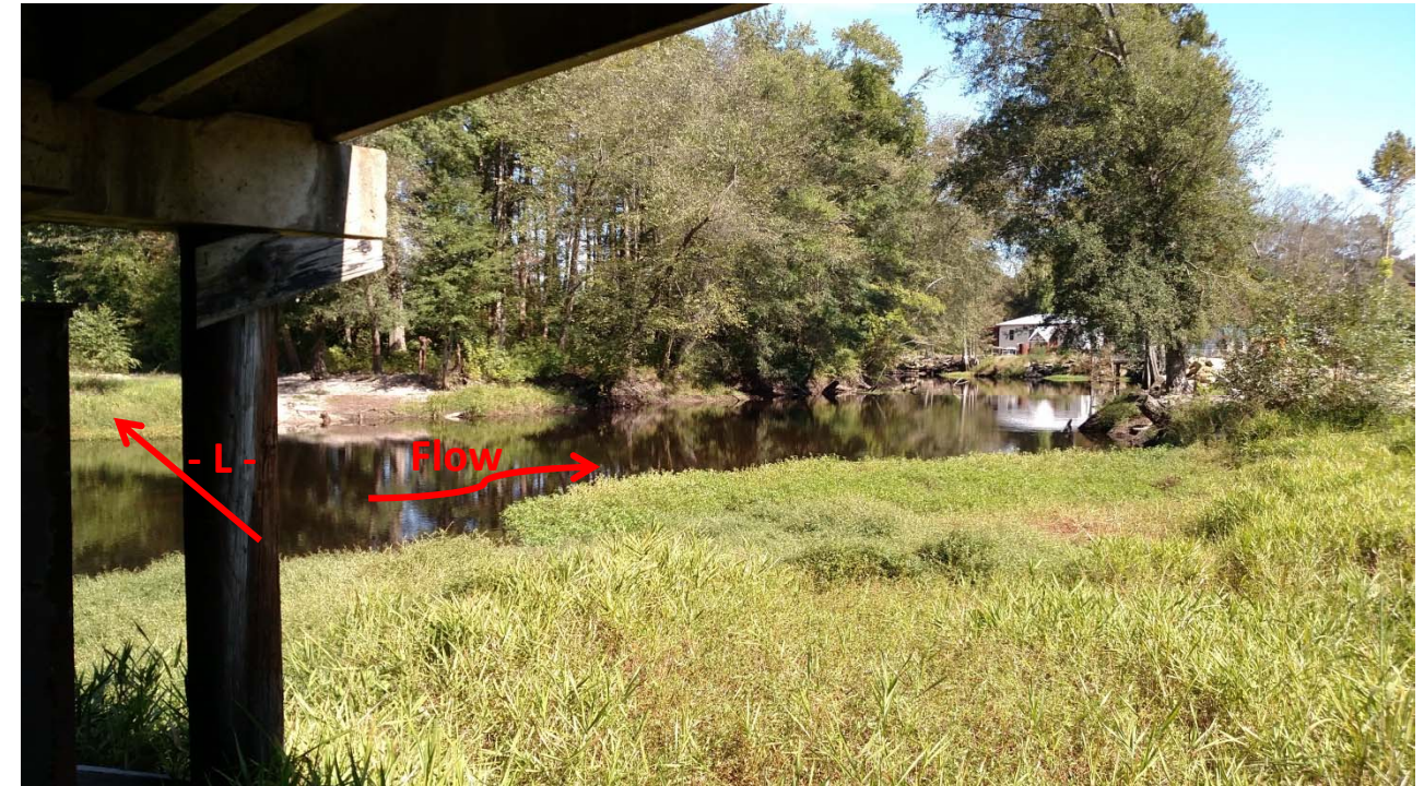
Photograph No. 3: View under the bridge looking downstream
