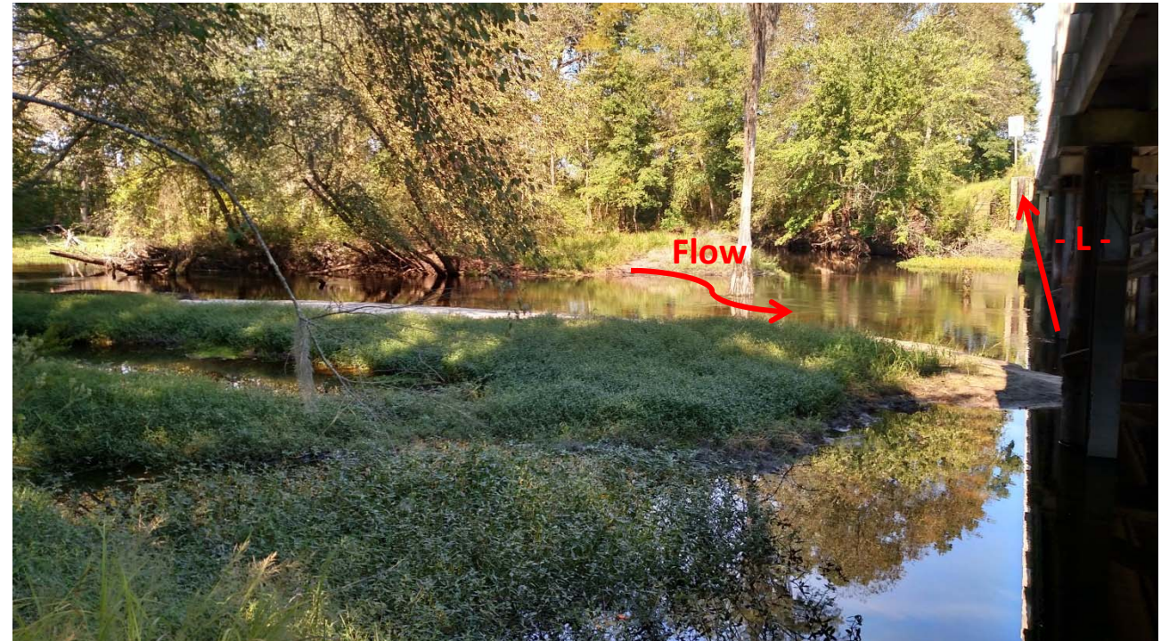
Photograph No. 4: View under the bridge looking northeast
