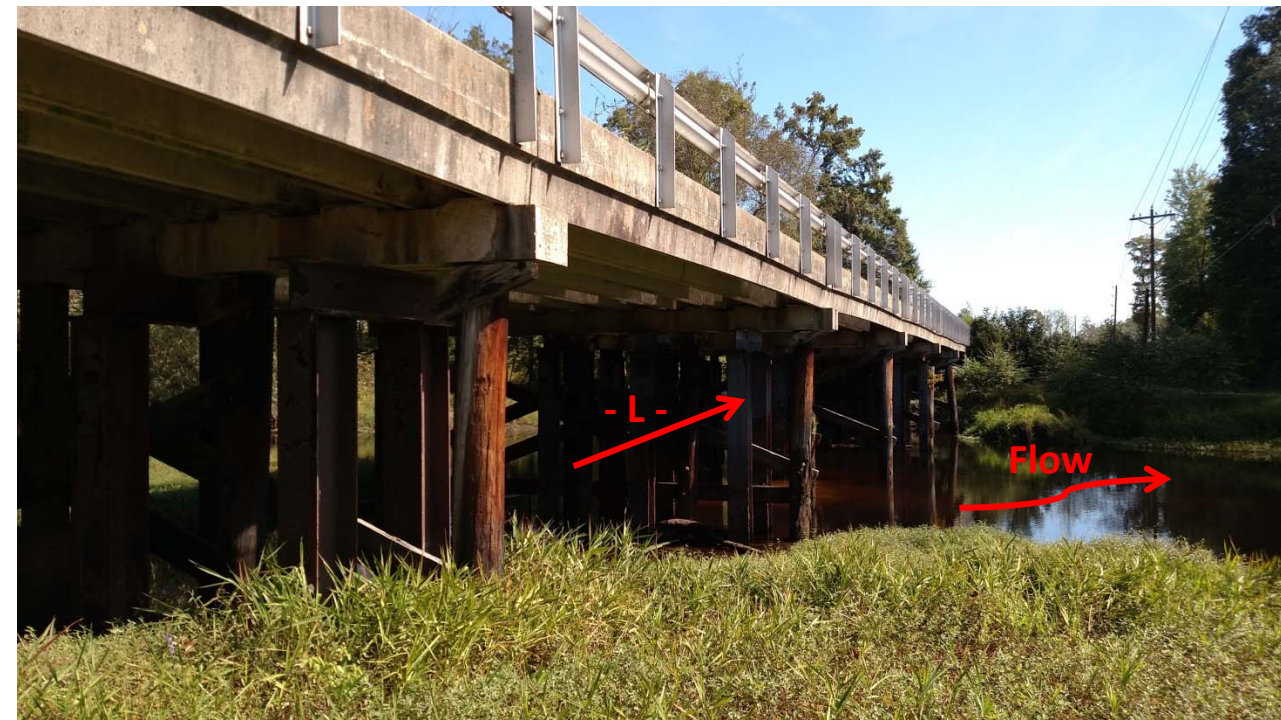
Photograph No. 2: View under the bridge looking northeast
