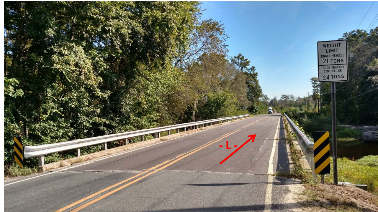
Photograph No. 1: View from End Bent 1 looking northeast
