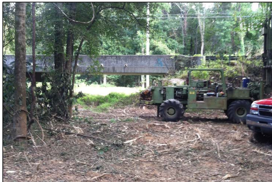
PHOTOGRAPH TAKEN FROM NEAR BORING EB1-C LOOKING TOWARD EXISTING STRUCTURE
