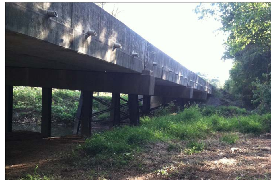
PHOTOGRAPH TAKEN FROM NEAR INTERIOR BENT 2 LOOKING DOWNSTATION TOWARD CHANNEL
