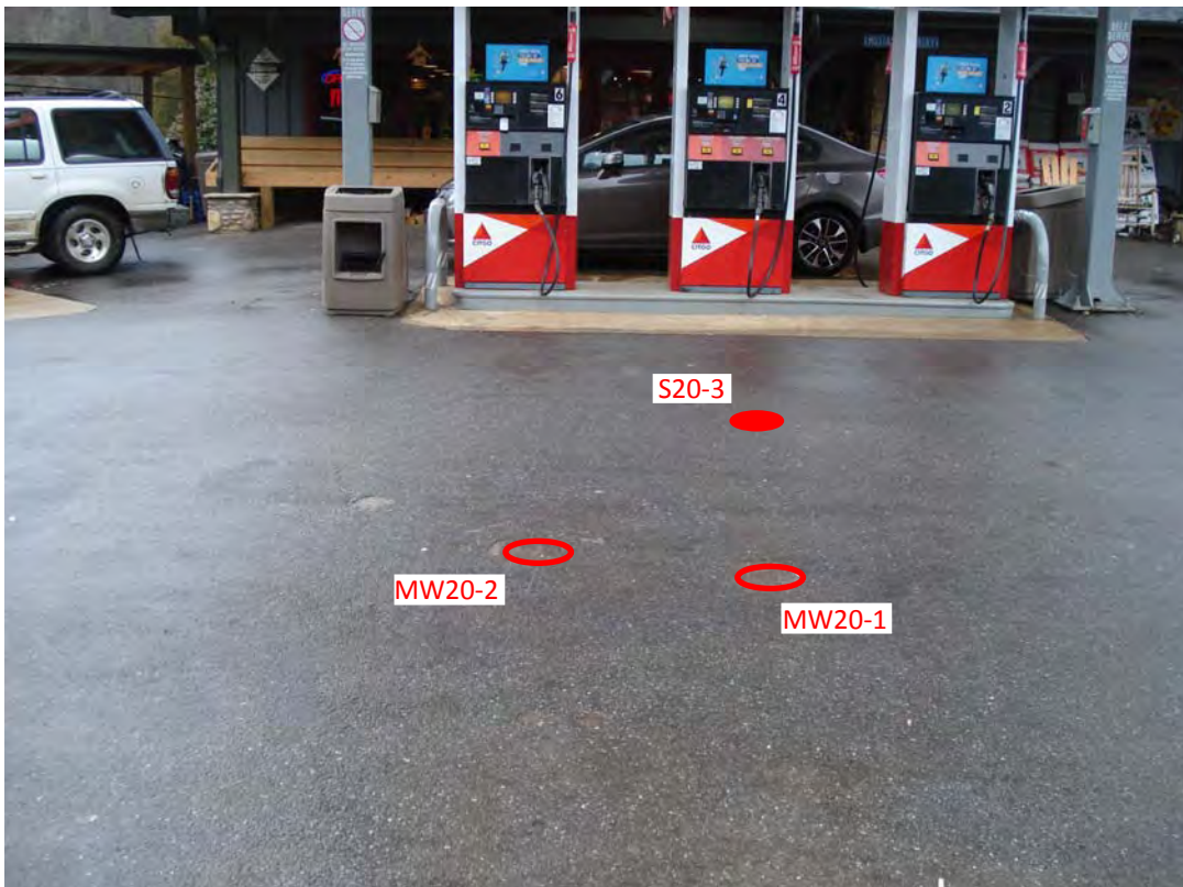
Photograph 4 : View looking west at locations of soil boring S20-3 and existing monitoring wells MW20-1 and MW20-2.
