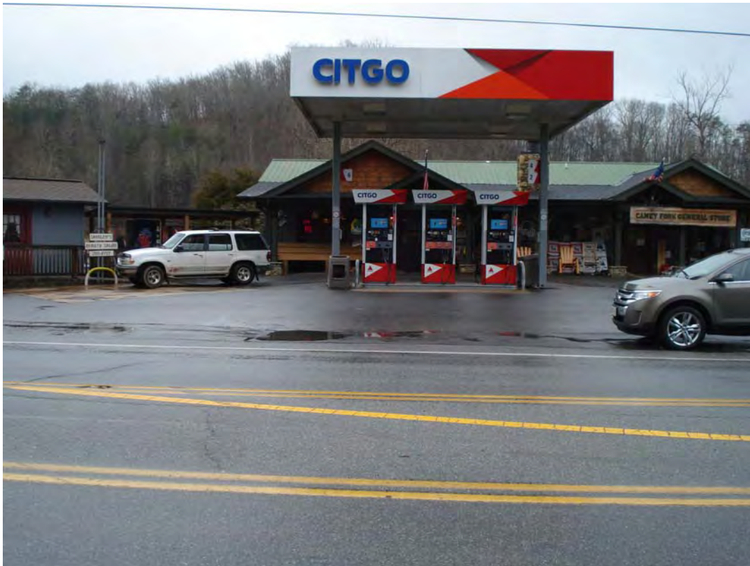
Photograph 1 : View looking west at Caney Fork General Store and Shirley's Beauty Salon (at left) on Parcel 020.
