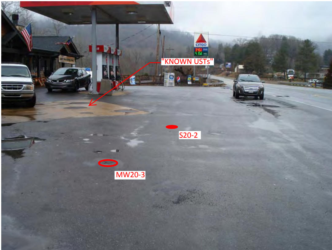
Photograph 3 : View looking south at locations of soil boring S20-2, existing monitoring well MW20-3, and "Known USTs."
