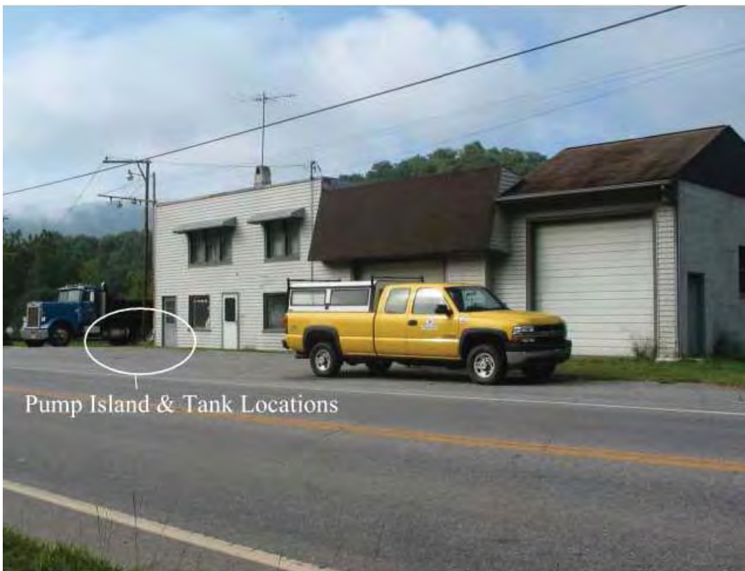
Photograph 6 : View looking south at closed service station in August 2006, prior to Demolition (photograph provided by NCDOT).
