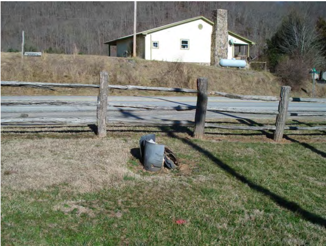
Photograph 5 : View looking east at abandoned water supply well.
