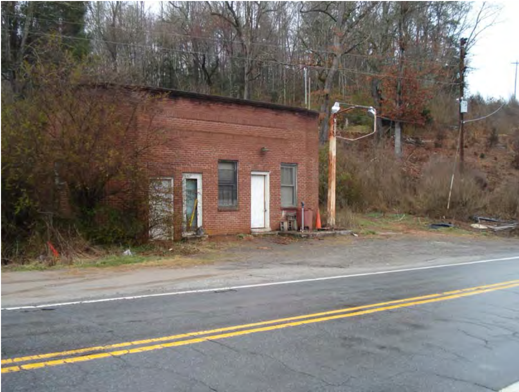
Photograph 1: View looking northeast at onsite structure. Former location of pump island is at concrete slab at east corner of building.
