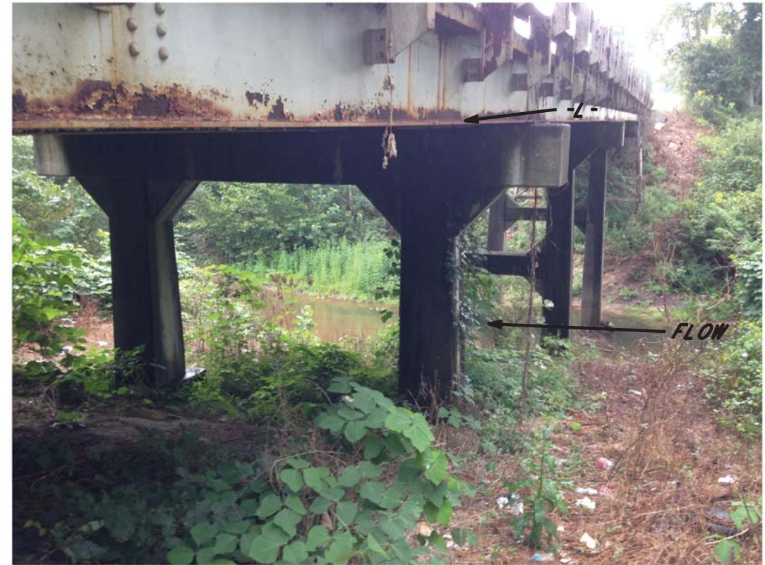
PHOTOGRAPH 2: VIEW UNDER BRIDGE 21 LOOKING SOUTH.
