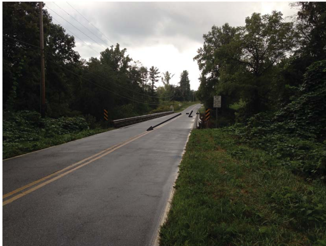
PHOTOGRAPH 1: VIEW OF JOHNSON BRIDGE RD. AT BRIDGE 21 LOOKING SOUTH.
