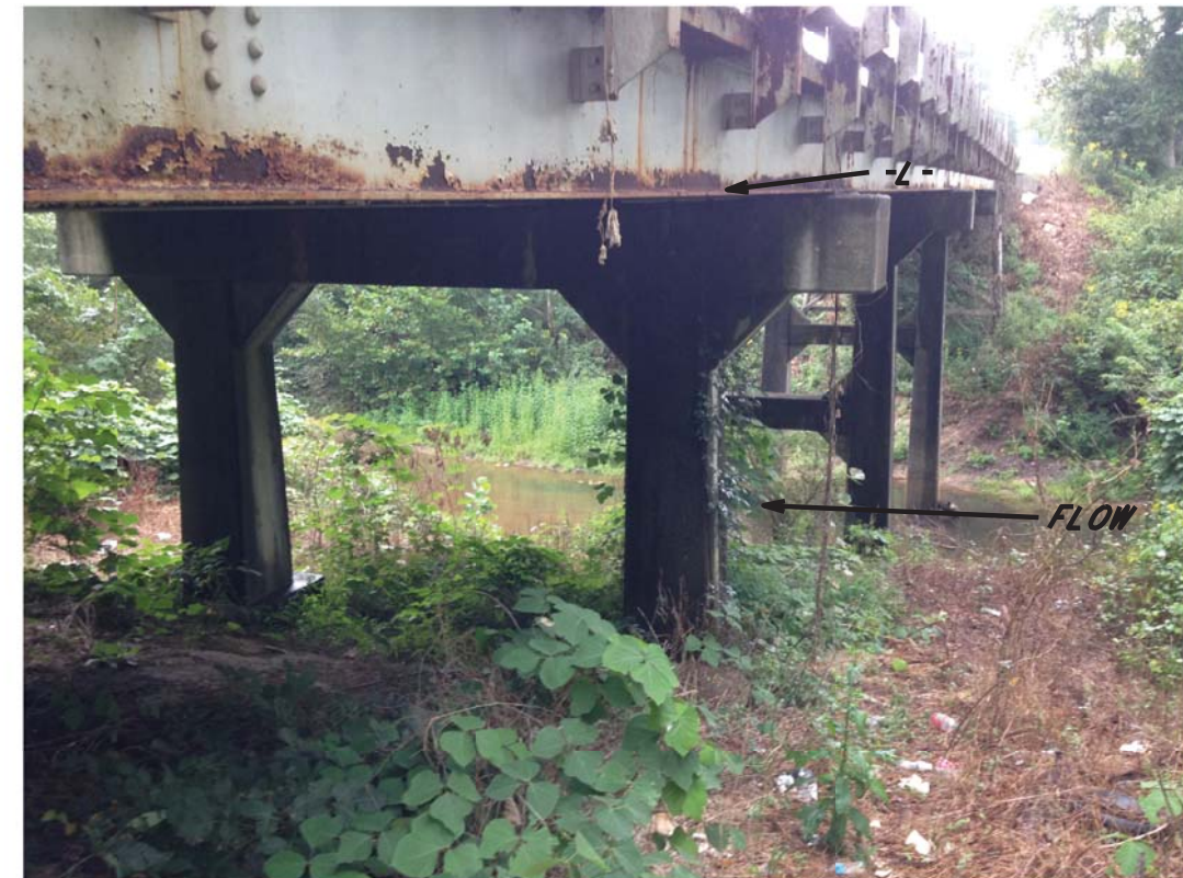
PHOTOGRAPH 2: VIEW UNDER BRIDGE 21 LOOKING SOUTH.
