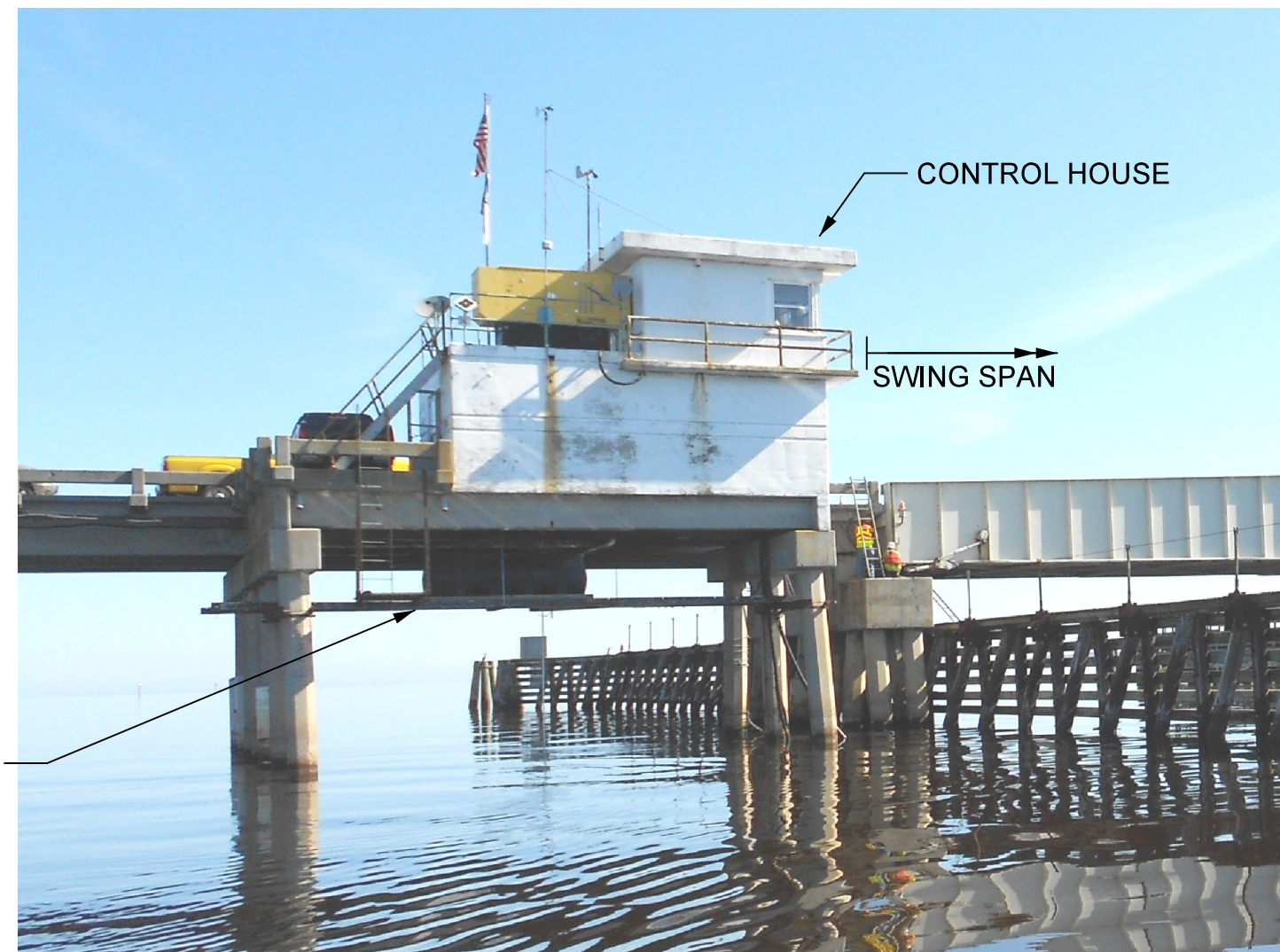
SEPTIC TANK PLATFORM
