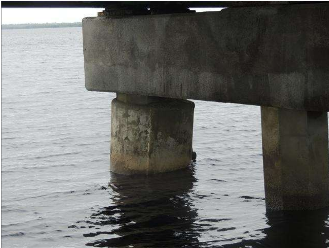
BENT 6 P4 HAS BEEN REPAIRED .
