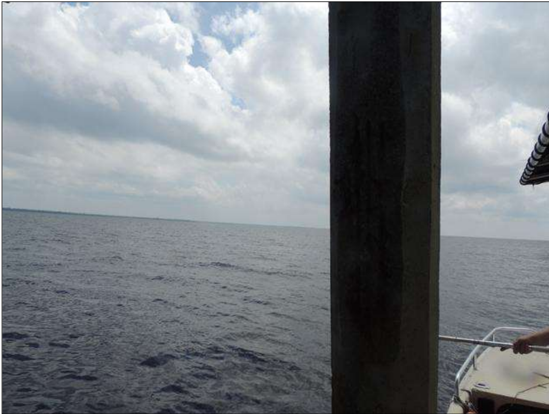
BENT 118 P5 CRACKED AND SPALLED AND DELAMINATED AREA WITH 5 CABLES EXPOSED 10' 10" H X 20" AROUND PILE.PM
