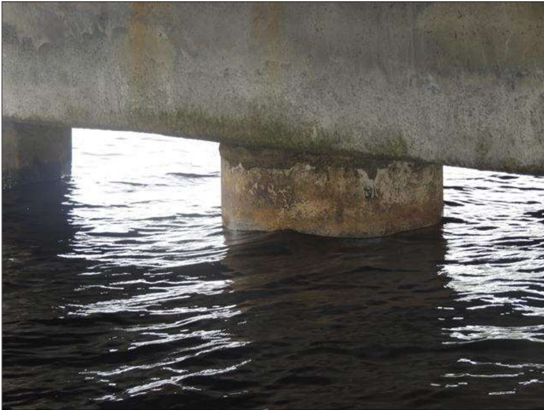
BENT 4 P3 HAS BEEN REPAIRED.
