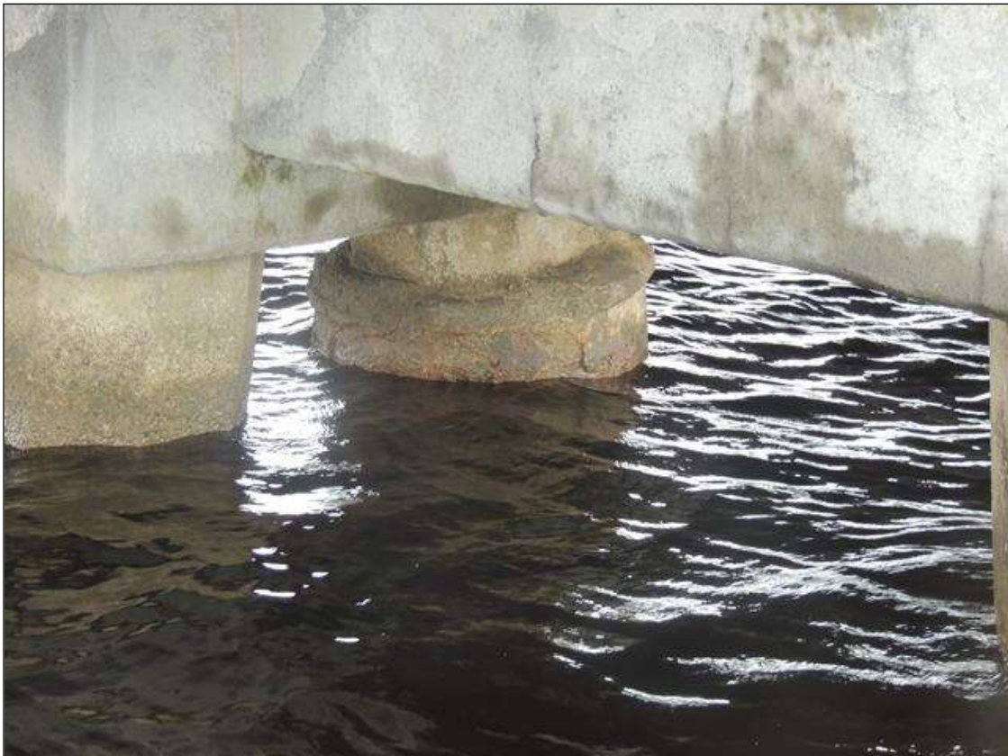
BENT 5 PILE 3 HAS BEEN REPAIRED.
