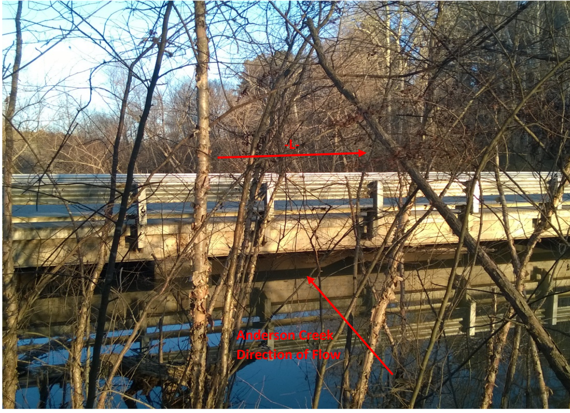
Profile of Bridge from South of End Bent 1
