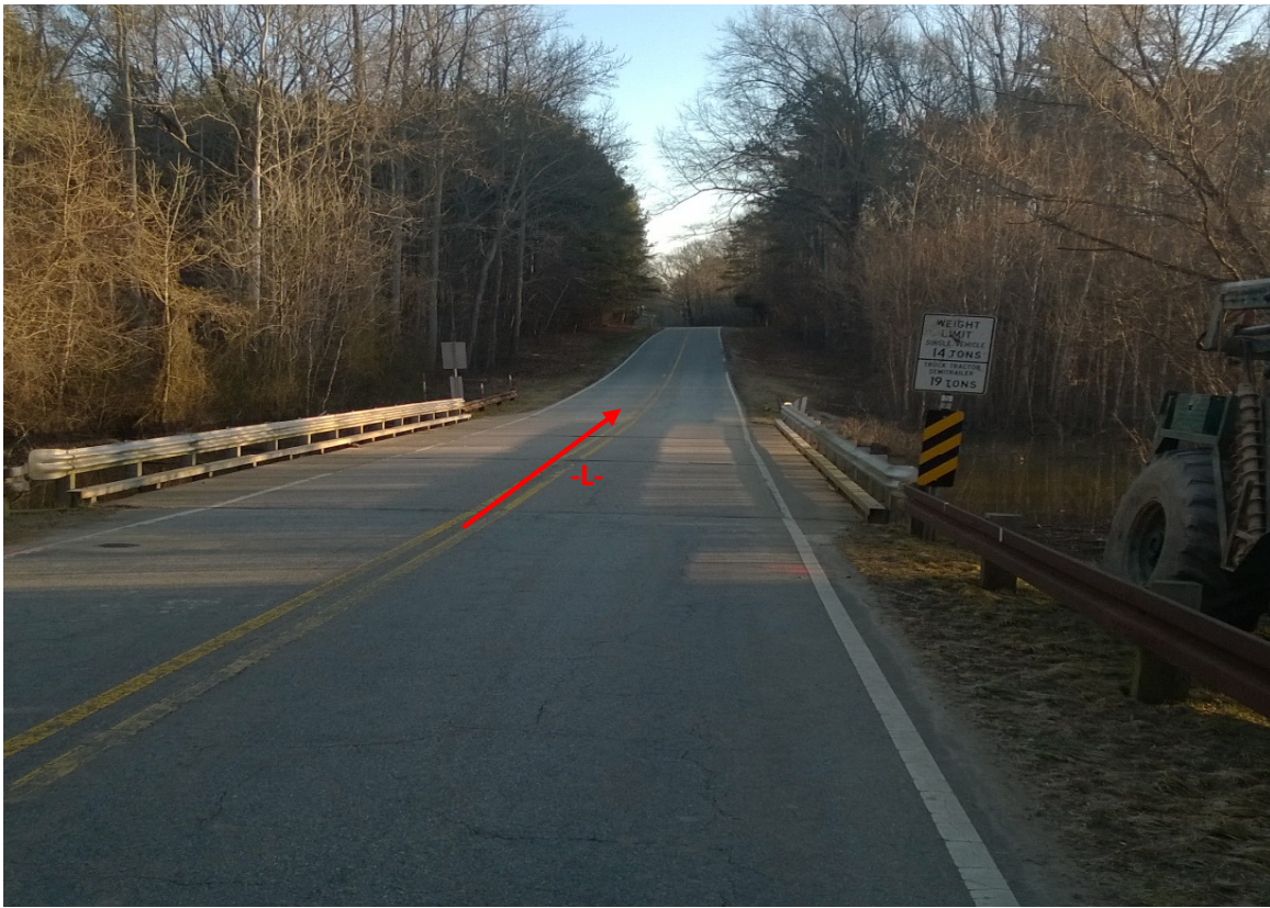
View Looking Northeast along -L- from End Bent 1
