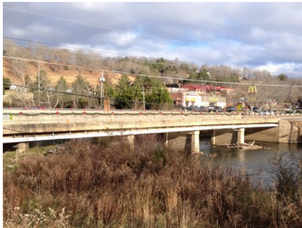
Photograph No. 3: This photograph was taken from the South side of the Little Tennessee River East of the US 441 -L- alignment, looking North
