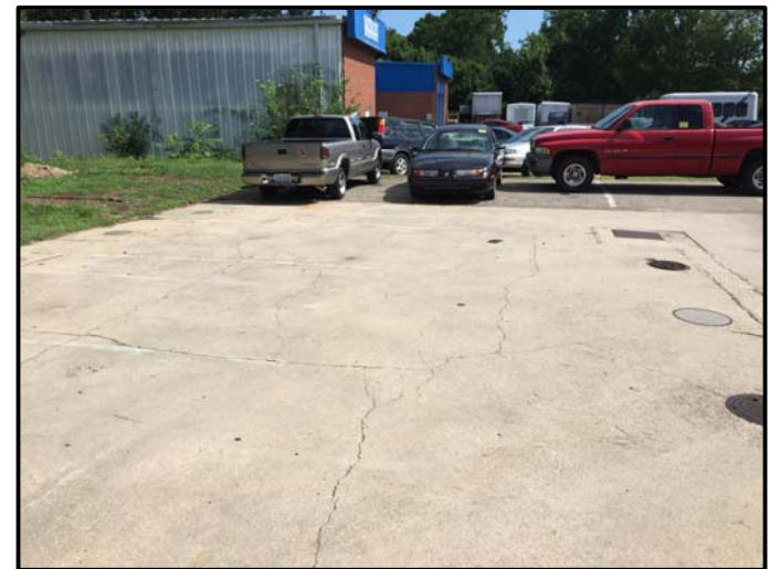
View of Supplemental Survey Area (Facing Approximately North)
