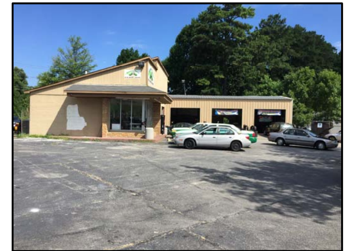
View of Survey Area (Facing Approximately West)
