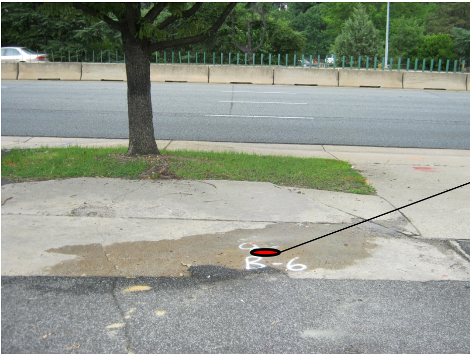
Photo #4: A view of Boring B-6, facing west.
