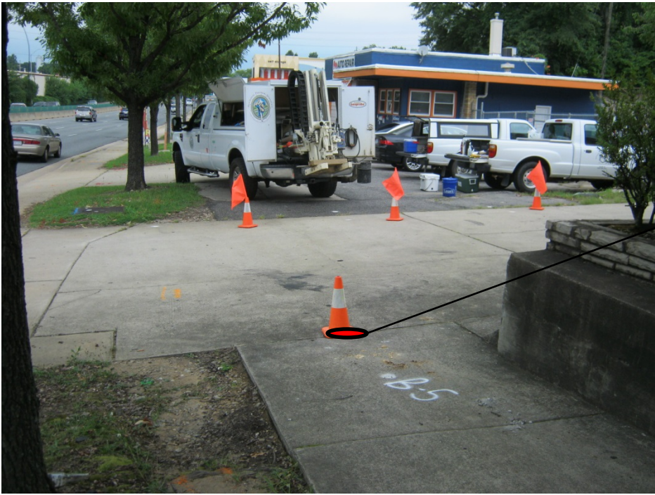
Photo #3: A view of boring location B-5, facing north.
