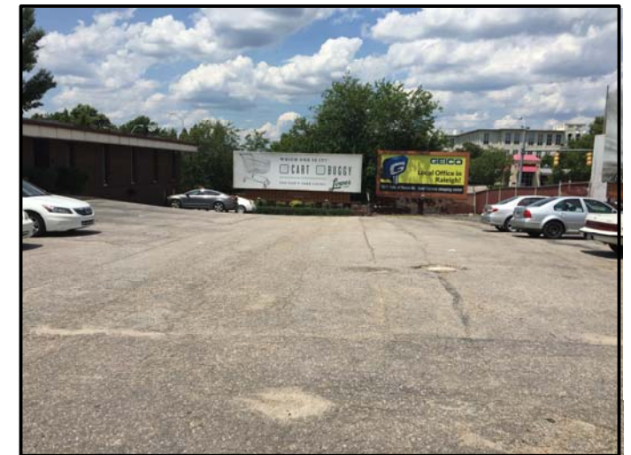
View of North Survey Area (Facing Approximately North)
