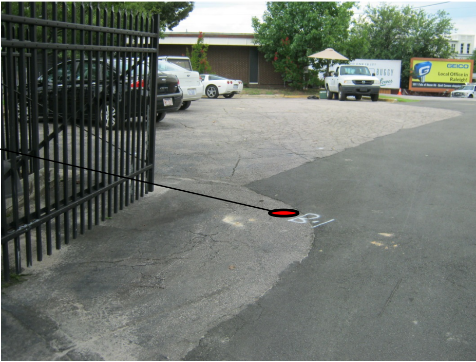
Photo #1: A view of boring location B-1, facing north.
