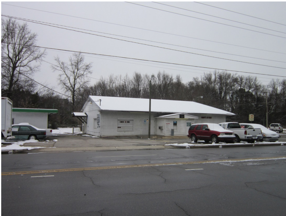
Parcel 11 (Utlely Rentals LLC Property), looking northeast
