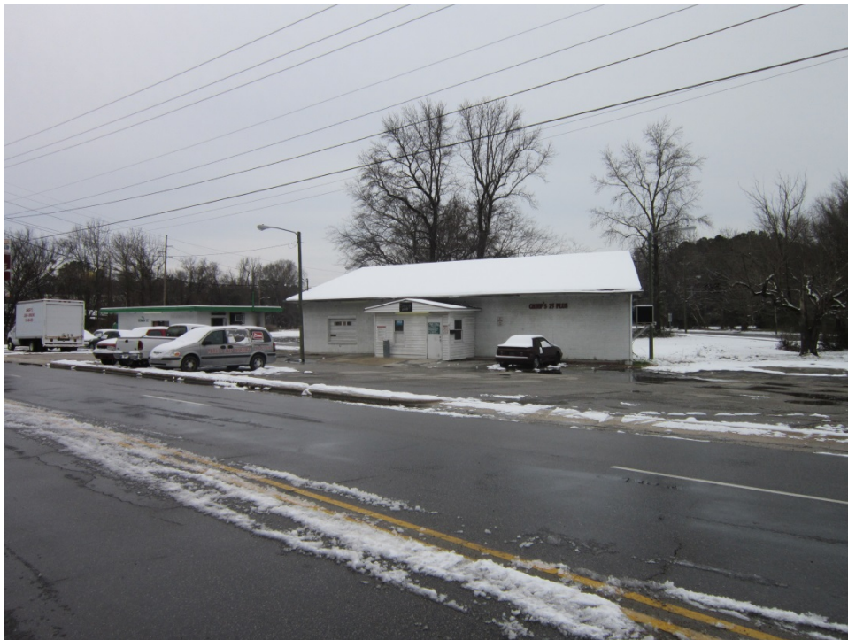
Parcel 11 (Utlely Rentals LLC Property), looking northwest
