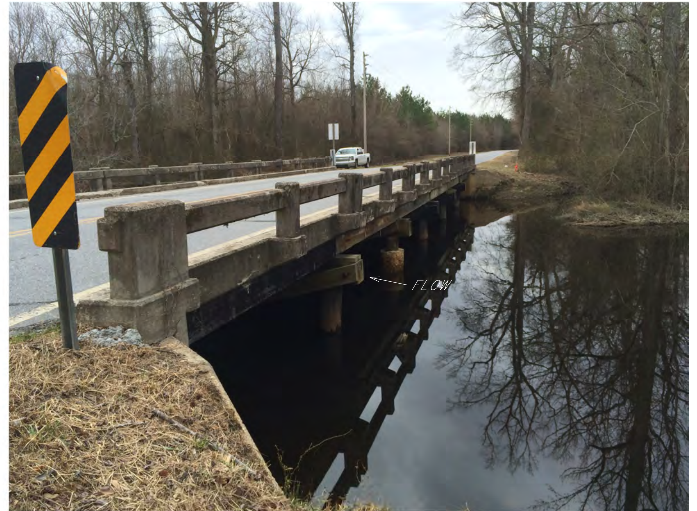
PHOTOGRAPH 2: VIEW LOOKING DOWNSTATION (SOUTH) ALONG -L- FROM END BENT 2.
