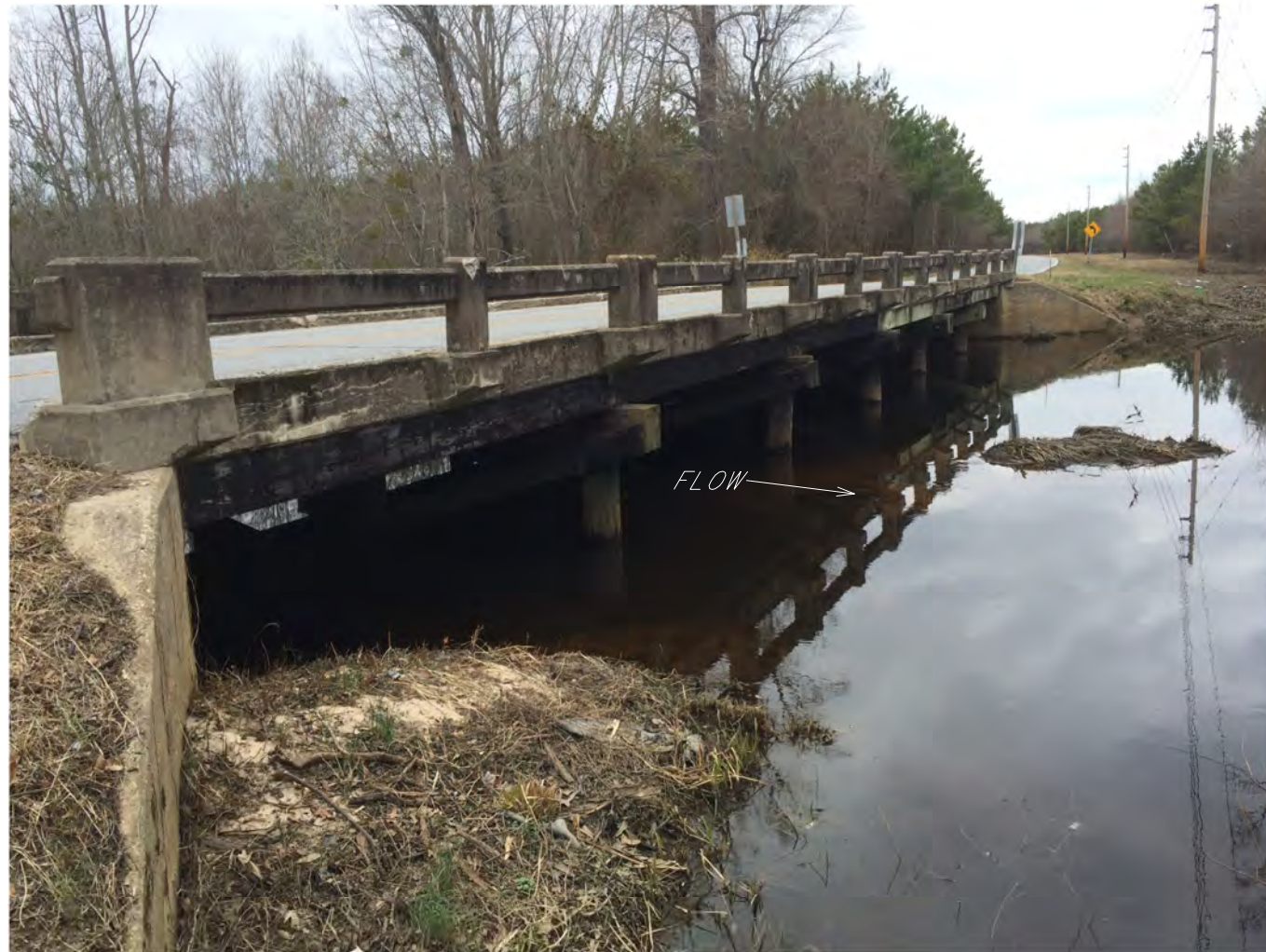
PHOTOGRAPH 1: VIEW LOOKING UPSTATION (NORTH) ALONG -L- FROM END BENT 1.
