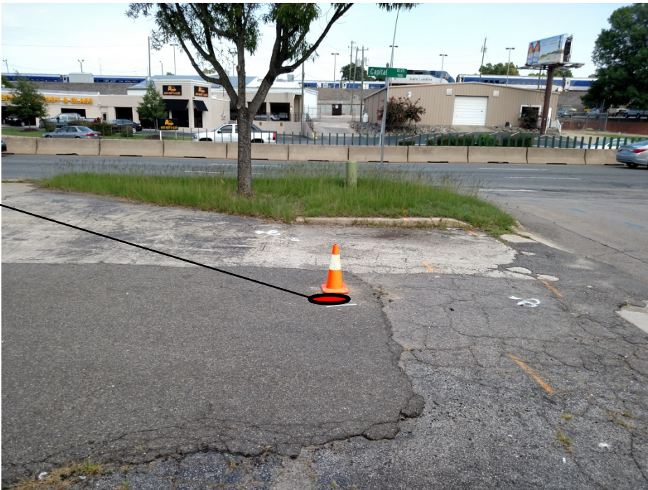
Photo #4: A view of Boring B-4, facing east.
