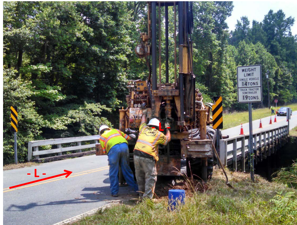
Photograph No. 1: View of drilling operations at boring EB1-B looking northwest
