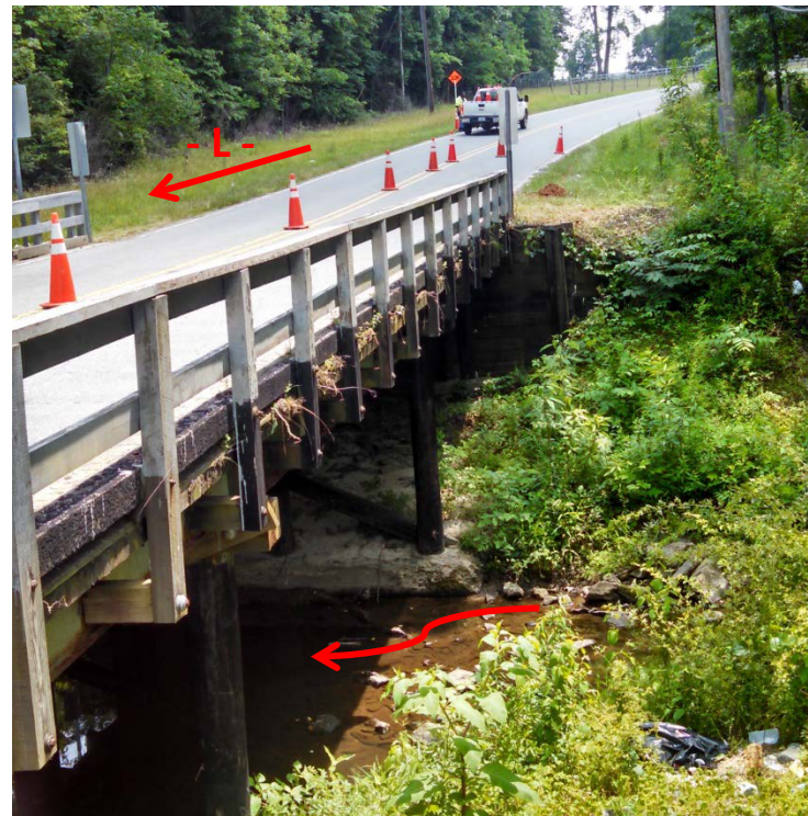
Photograph No. 2: View of End Bent 1 looking south
