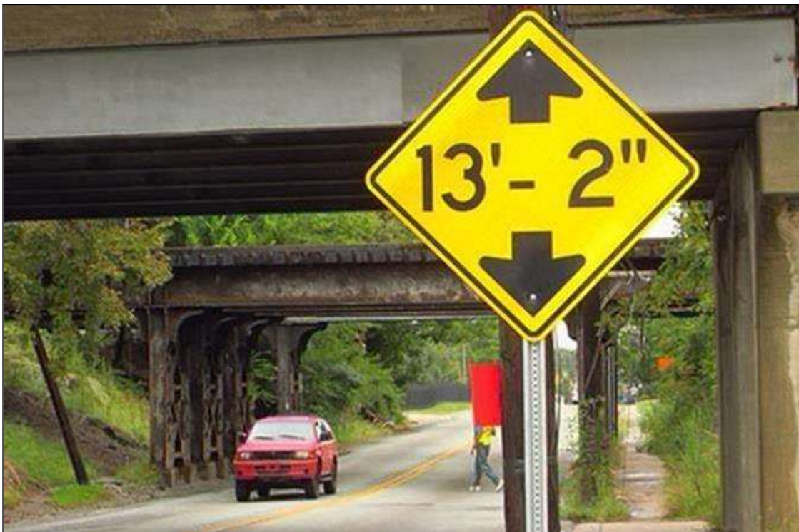
CLEARANCE SIGN ON EAST SIDE
