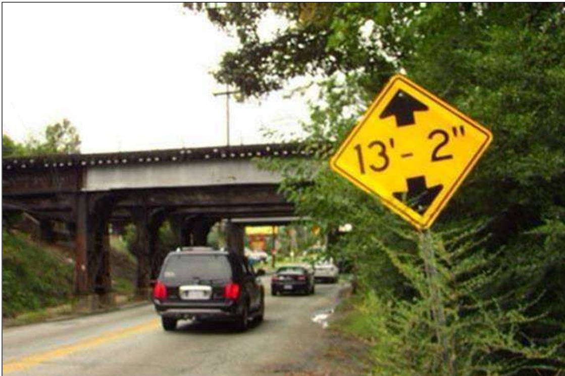
EAST SIDE CLEARANCE SIGN
