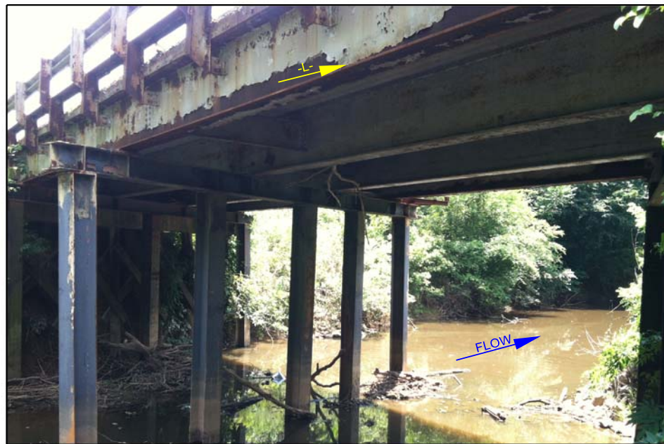
PHOTOGRAPH TAKEN FROM EAST OF END BENT 2 LOOKING LEFT AND SHOWING EXISTING INTERIOR BENTS
